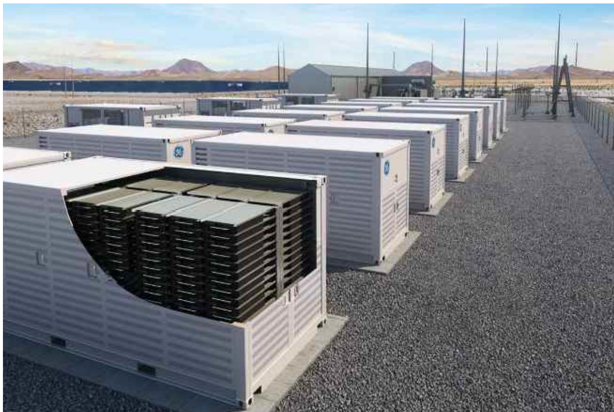
Figure 3-3: Typical BESS Arrangement
