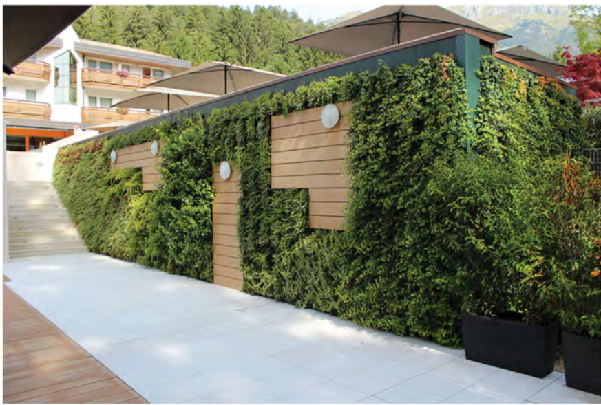
Green wall with panel
