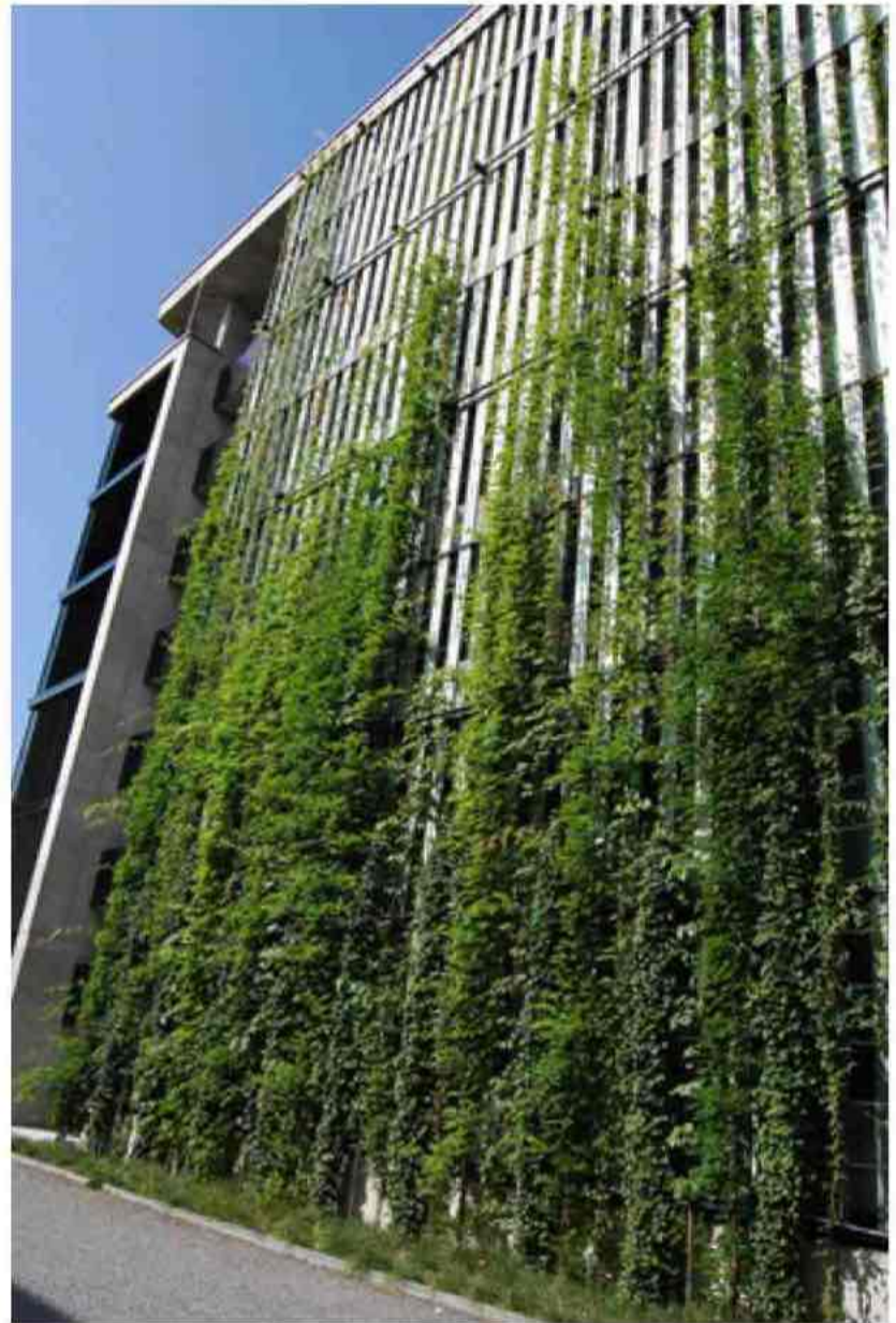
Green trellis climbers on facade
