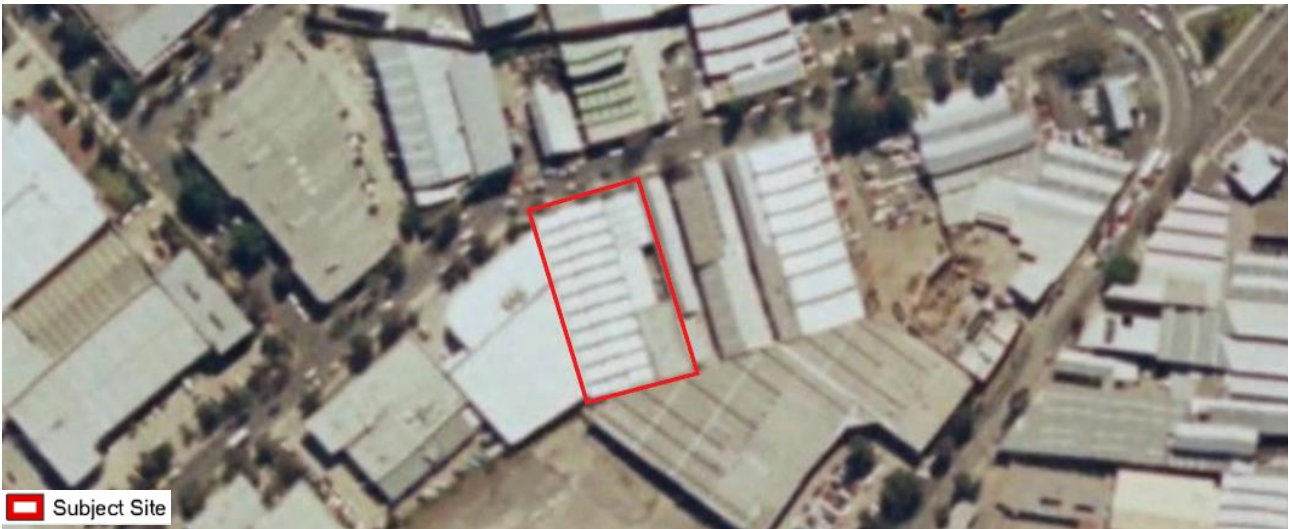
Figure 17 – Detail from 2004 aerial, showing buildings on subject site – note new roof cladding to all buildings Source: NSW Spatial Services, Historical Imagery, with Urbis overlay
