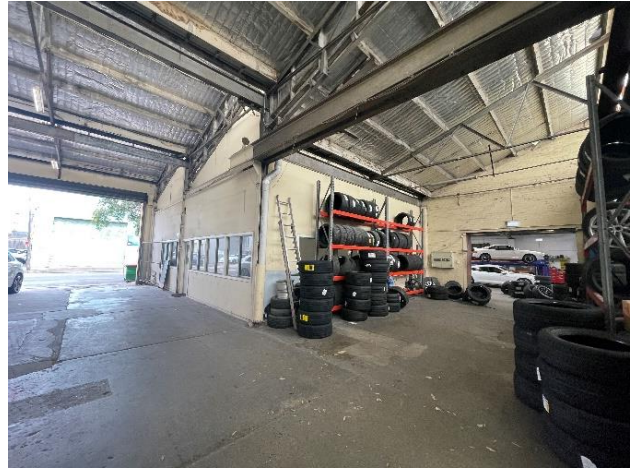
Figure 23 – Lightweight partitions creating office space in no. 30-32
