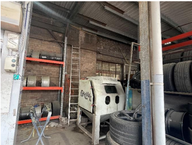
Figure 24 – Detail of eastern wall to building at no. 30-32
