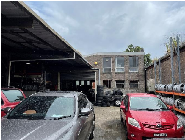
Figure 26 – Rear of the front building at no. 28
