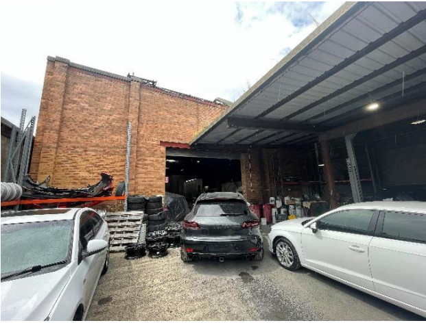
Figure 28 – Entrance to rear building at no. 28, from the breezeway
