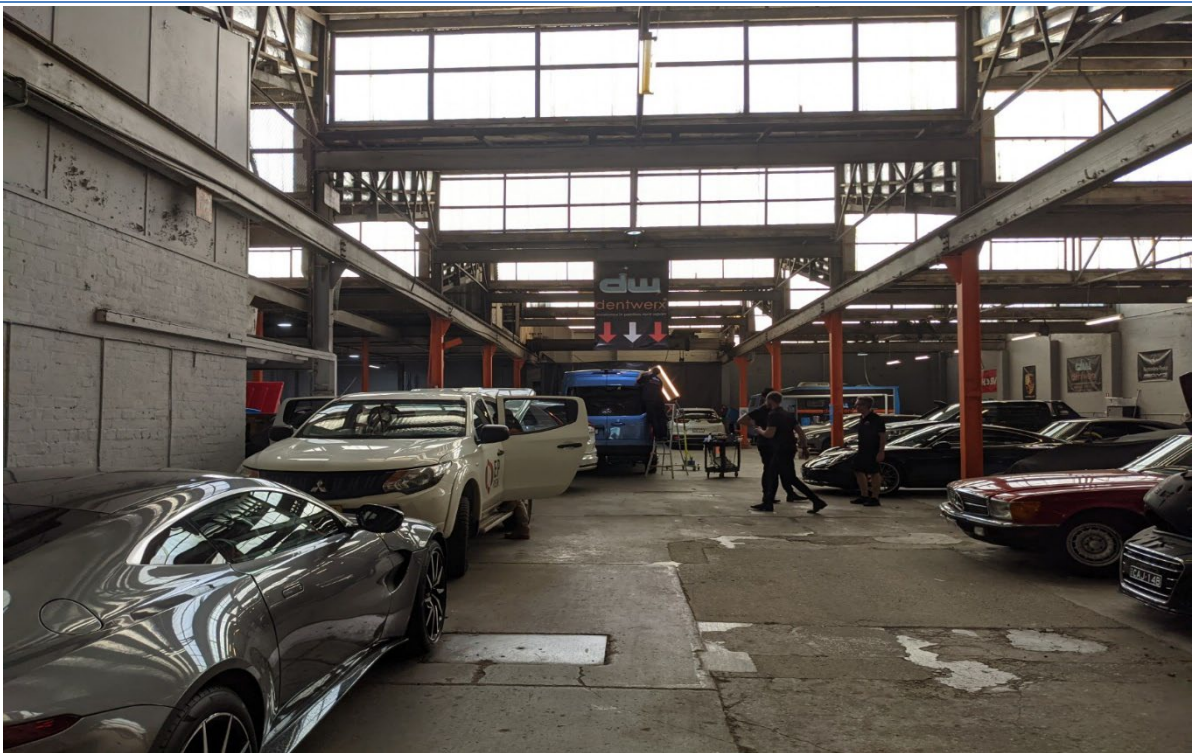
Plate 2 – Eastern portion of warehouse, facing south, concrete slab observed throughout the Site.
