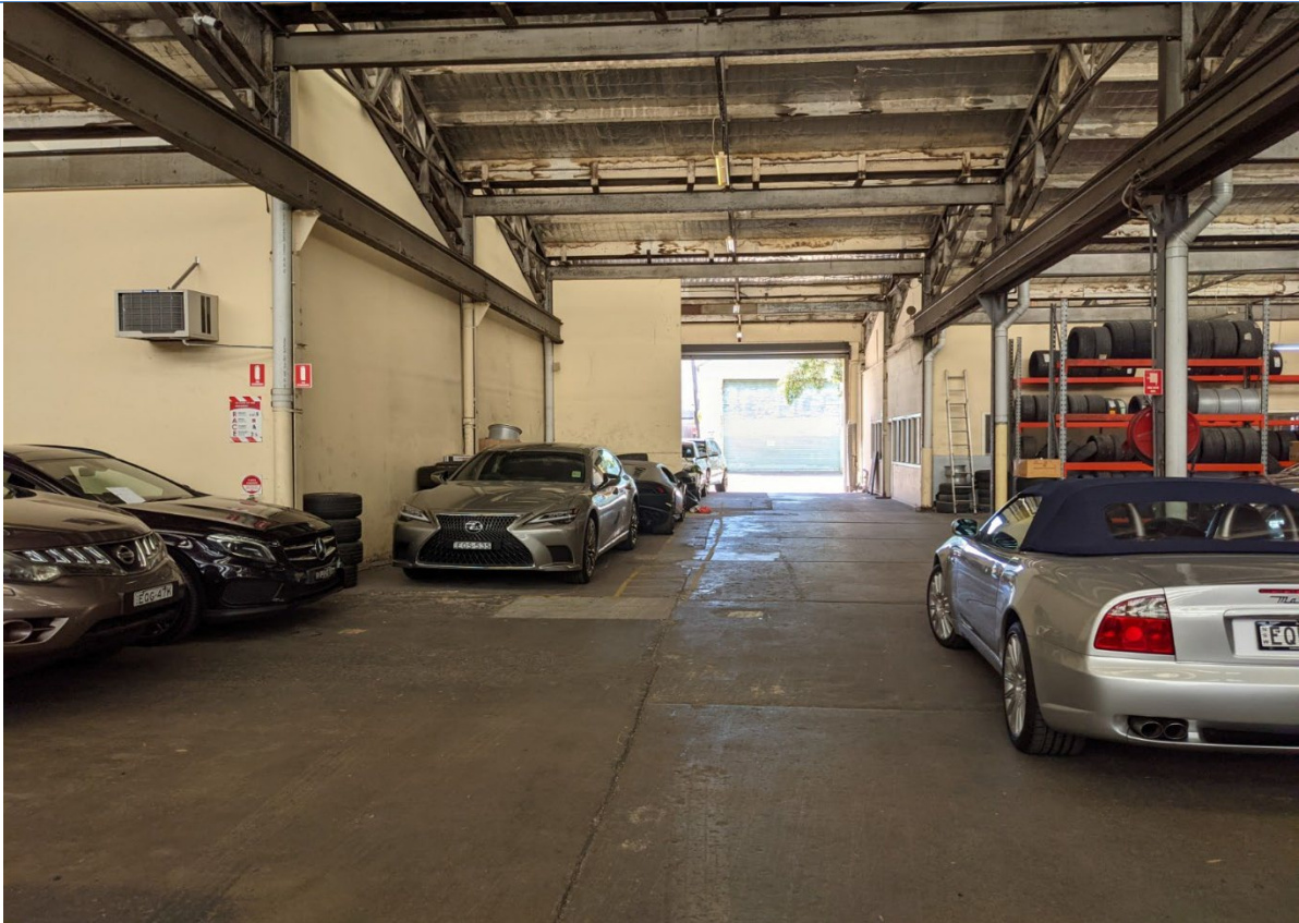
Plate 1 – Eastern portion of warehouse, facing north, concrete, slab observed throughout the Site.
