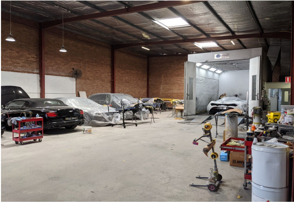
Plate 3 – Western Portion of warehouse, south extent, facing south, concrete, slab observed throughout the Site.
