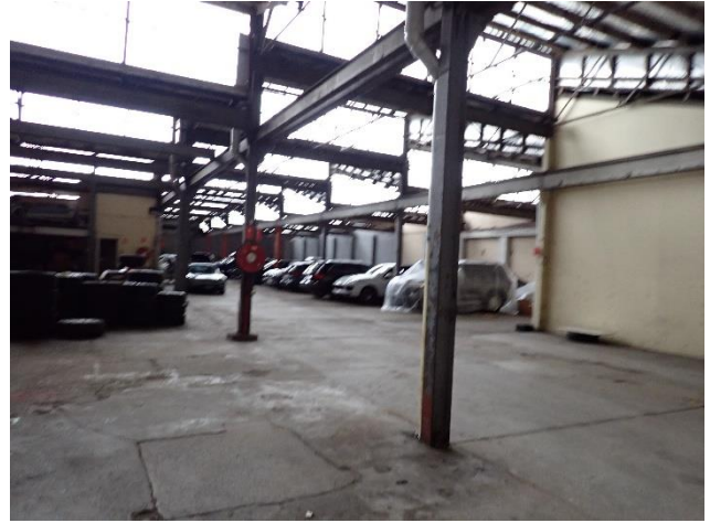
Figure 23- Interior of building.
