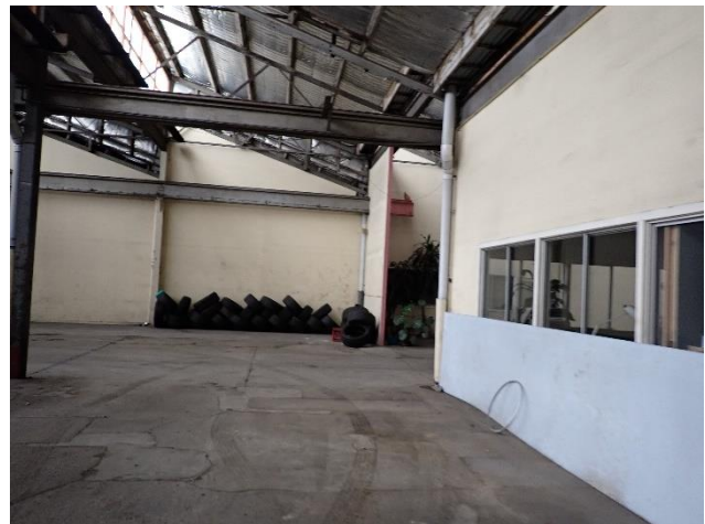
Figure 19- Inside the building showing concrete floor.
