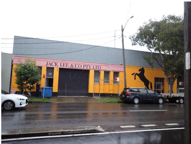
Figure 18- Front of building from Bourke Street.
