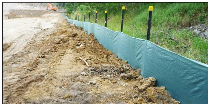
Figure 4: Sediment Fence
