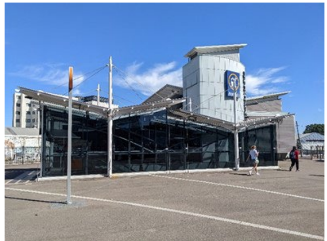
Picture 6 View of entry to Green Square Station
