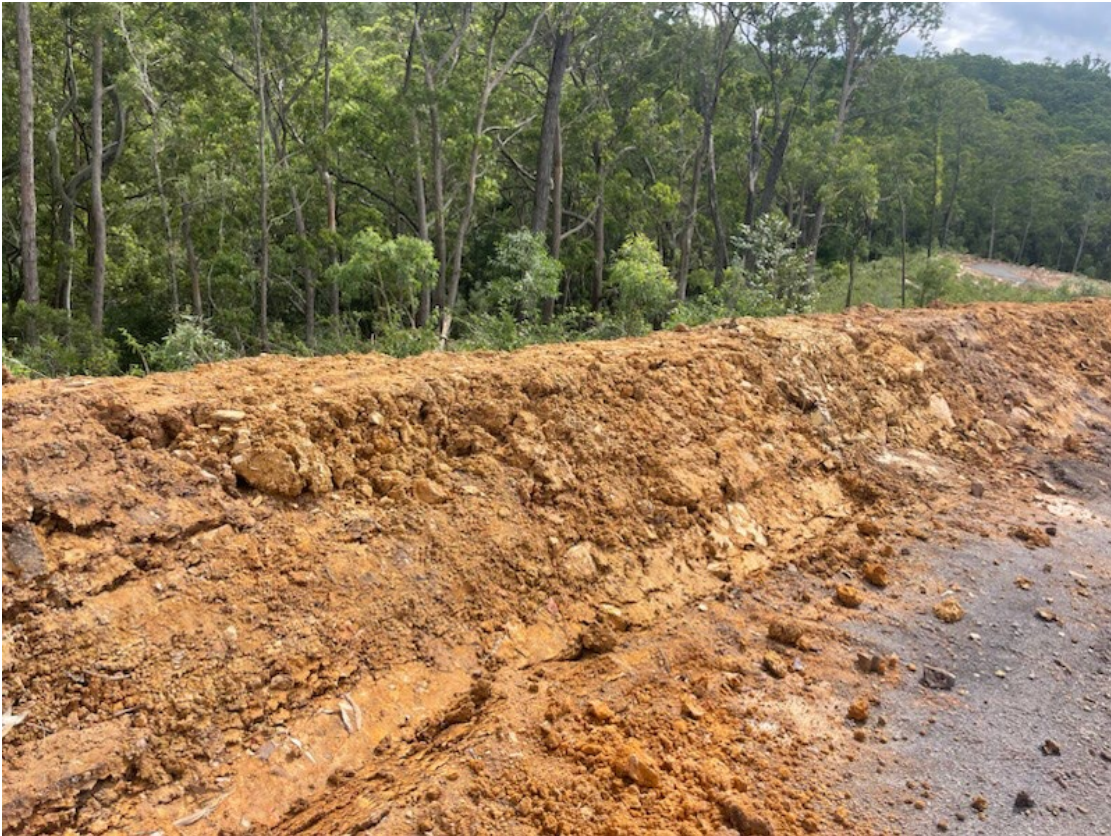
Clean Water Division Bund – Southern Side of Stage 1.
