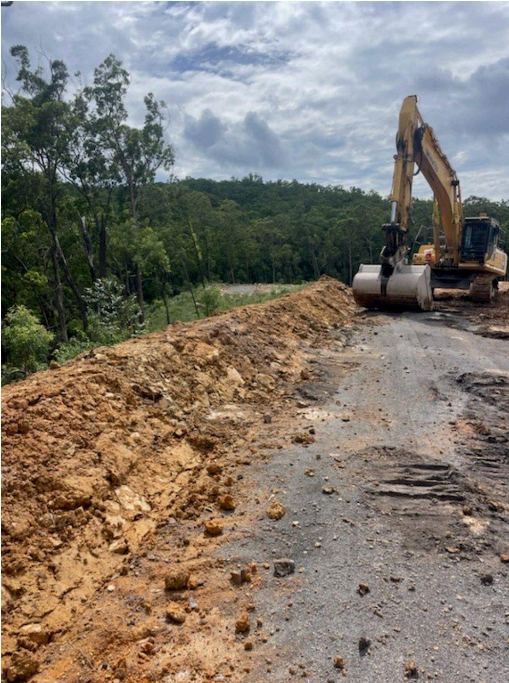
Clean Water Division Bund – Southern Side of Stage 1.
