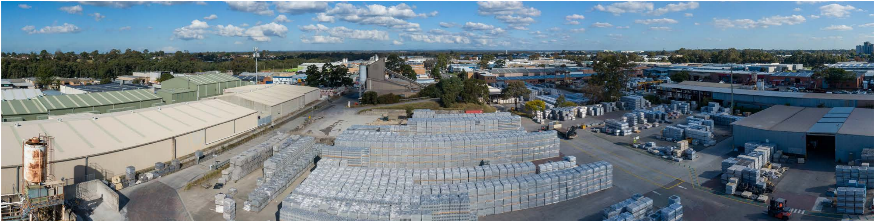
Figure 5: Drone at Position 1 - Looking South (May 2023)
