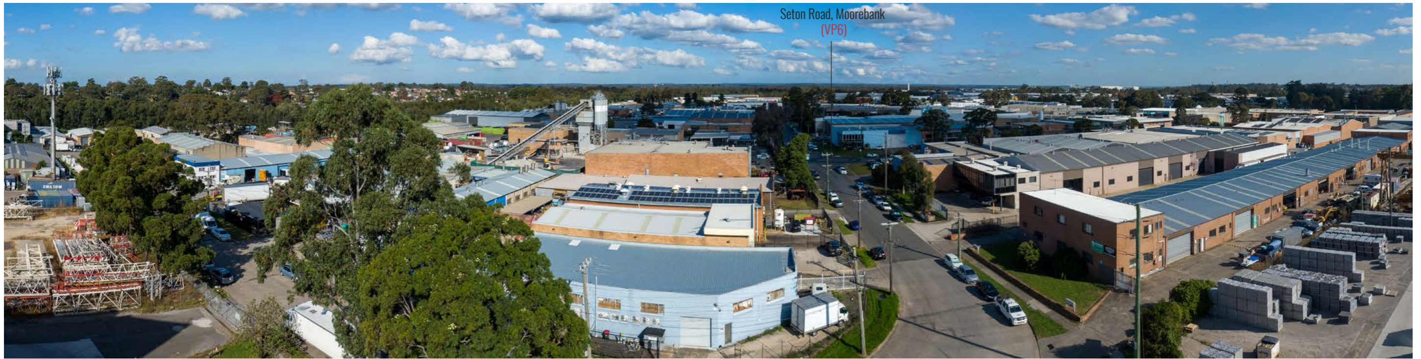
Figure 13: Drone at Position 3 - Looking South (May 2023)
