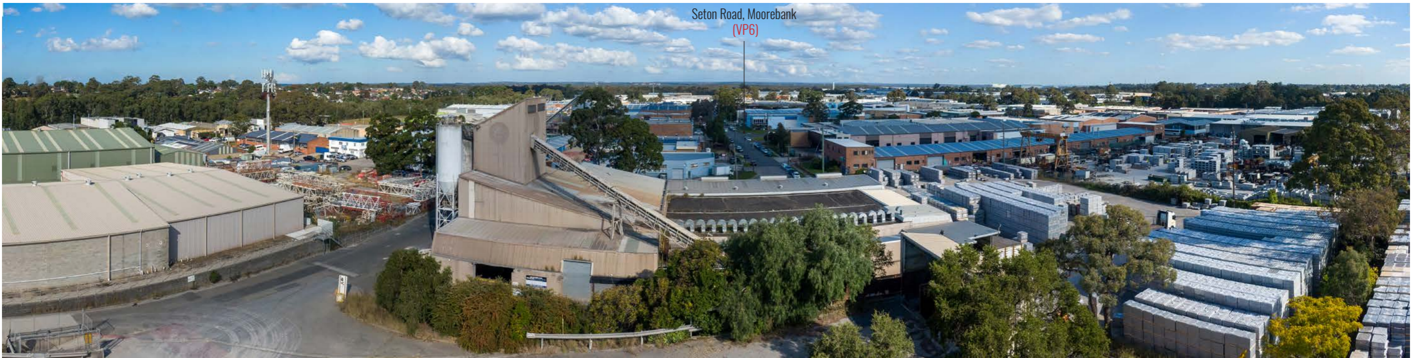
Figure 9: Drone at Position 2 - Looking South (May 2023)
