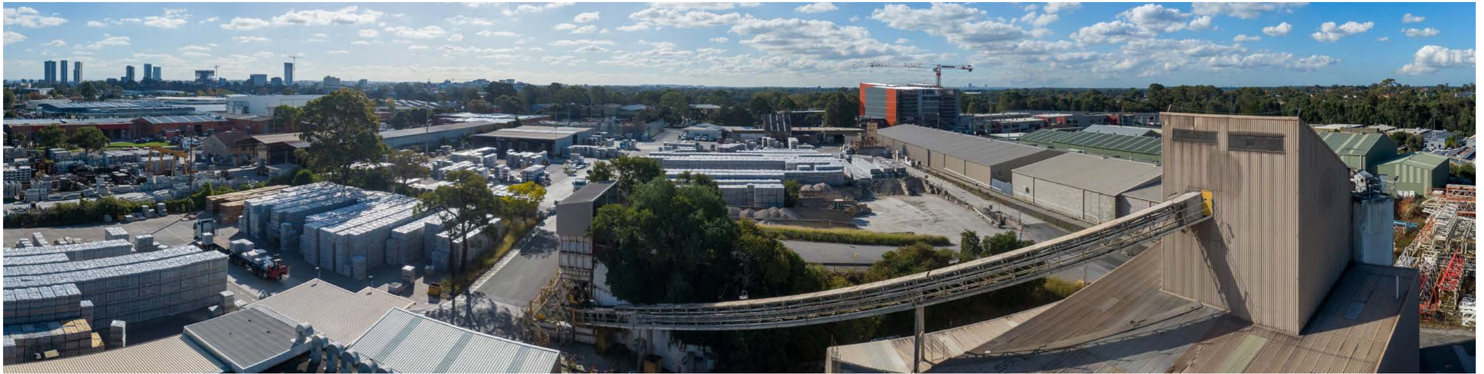
Figure 11: Drone at Position 3 - Looking North (May 2023)
