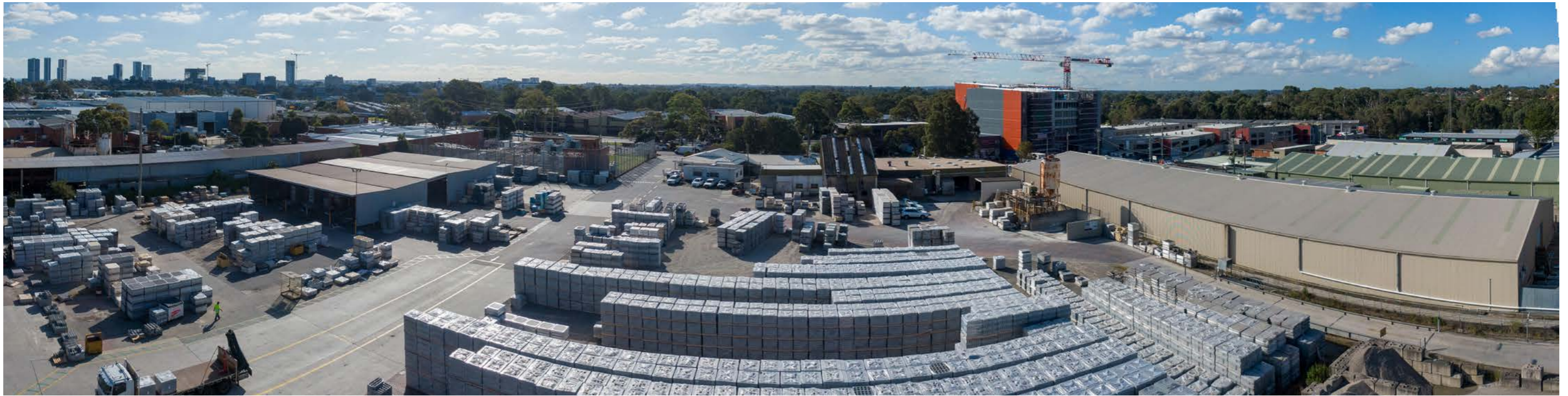
Figure 7: Drone at Position 2 - Looking North (May 2023)
