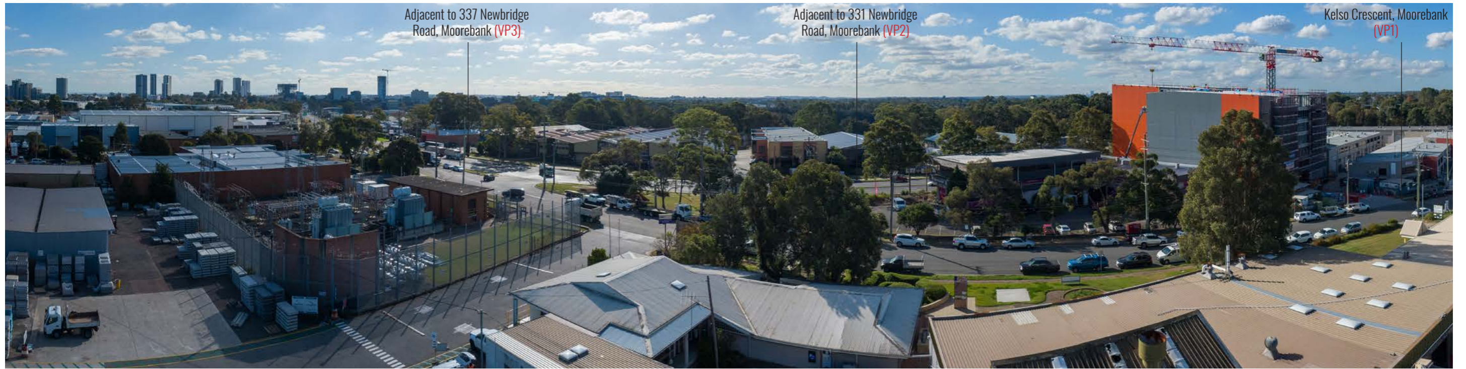
Figure 3: Drone at Position 1 - Looking North (May 2023)
