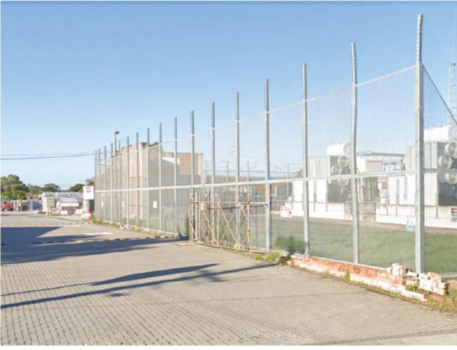
IMAGE --FENCE TYPE 3 --EXISTING AT 24 KELSO CR SUBSTATION
