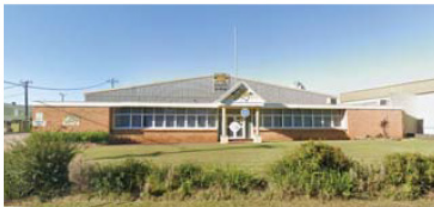
18 Kelso Crescent - E4 General Industrial
