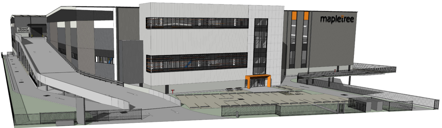
NORTH-EAST VIEW FROM KELSO CRESCENT
