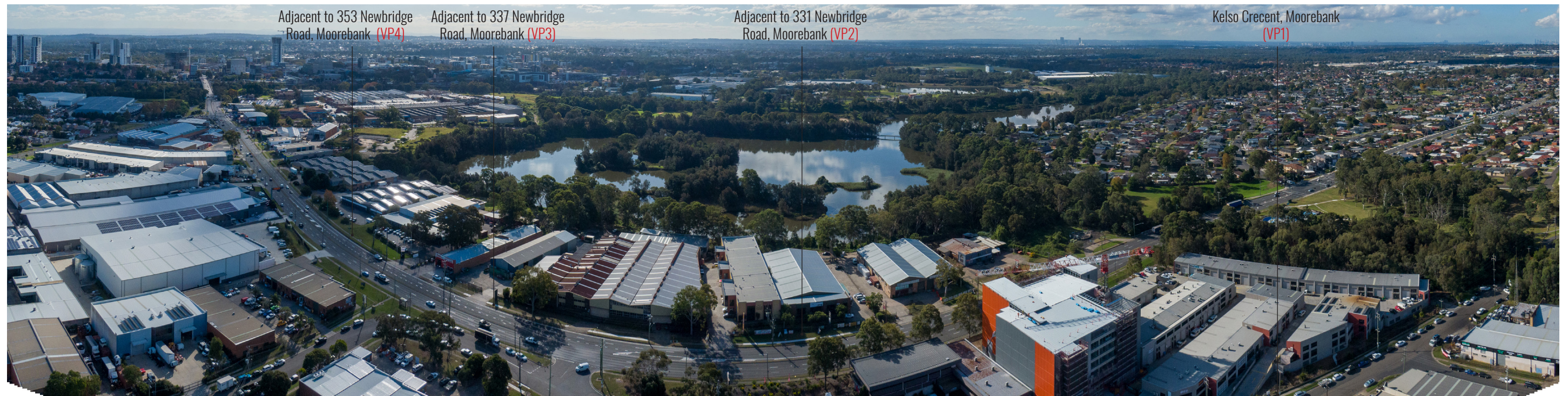
Figure 15: Drone at Position 2 - 120m AGL - Looking North
