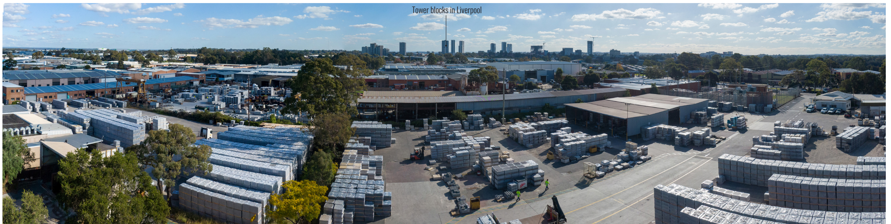
Figure 10: Drone at Position 2 - RL 35.1m - Looking West
