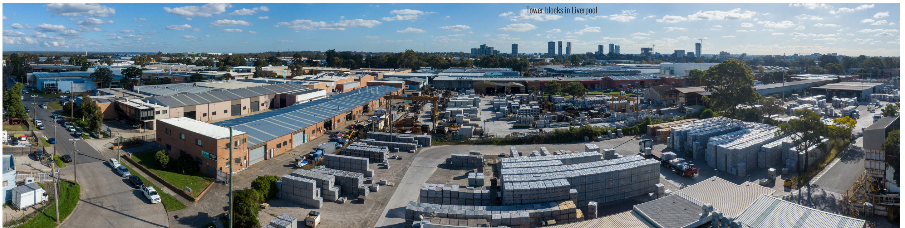
Figure 14: Drone at Position 3 - RL 35.1m - Looking West
