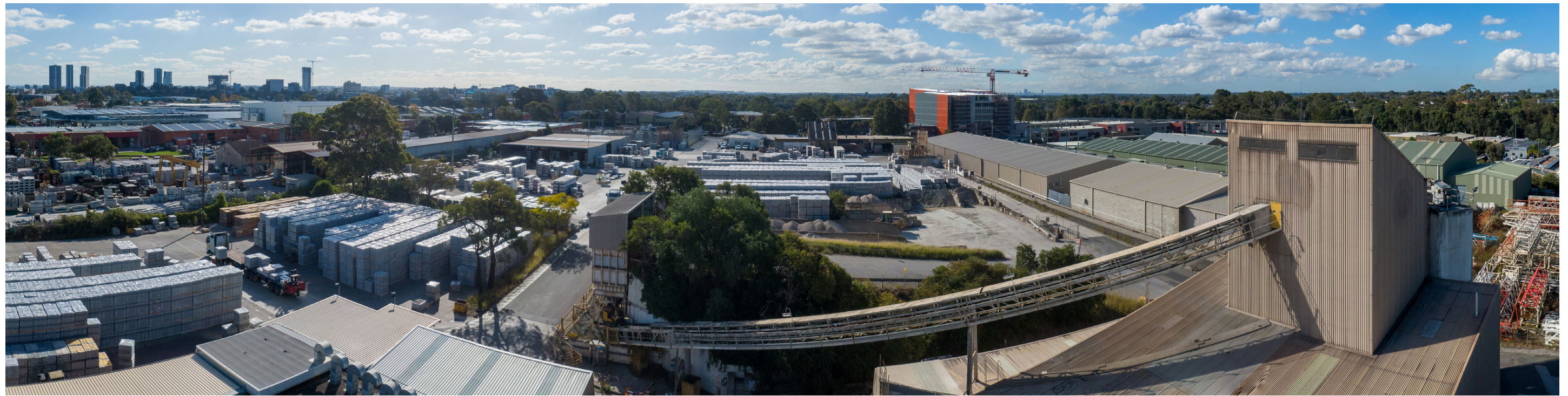
Figure 11: Drone at Position 3 - RL 35.1m - Looking North
