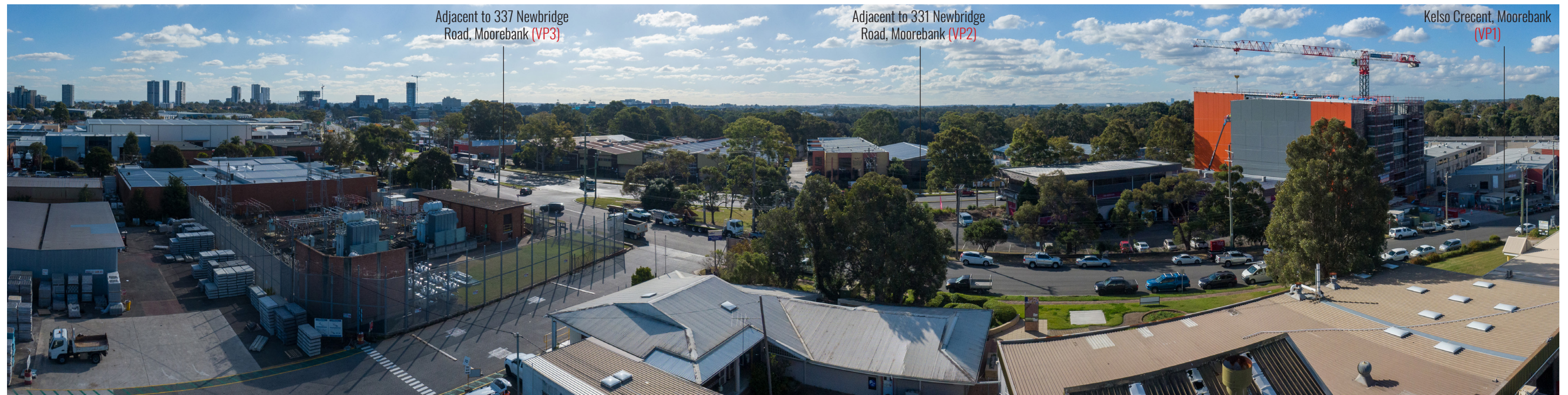
Figure 3: Drone at Position 1 - RL 35.1m - Looking North
