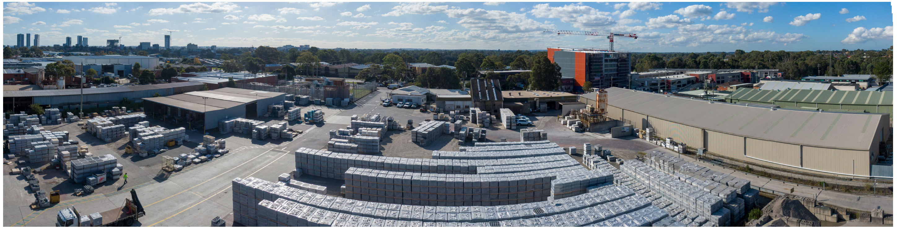
Figure 7: Drone at Position 2 - RL 35.1m - Looking North
