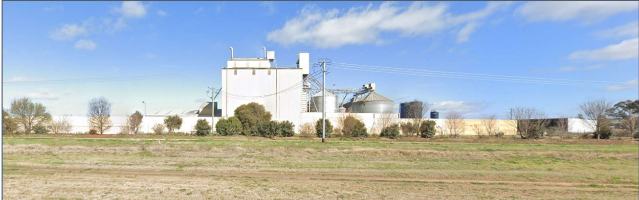
Figure 5: Photograph of Existing Mill (Google Maps, 2024)
