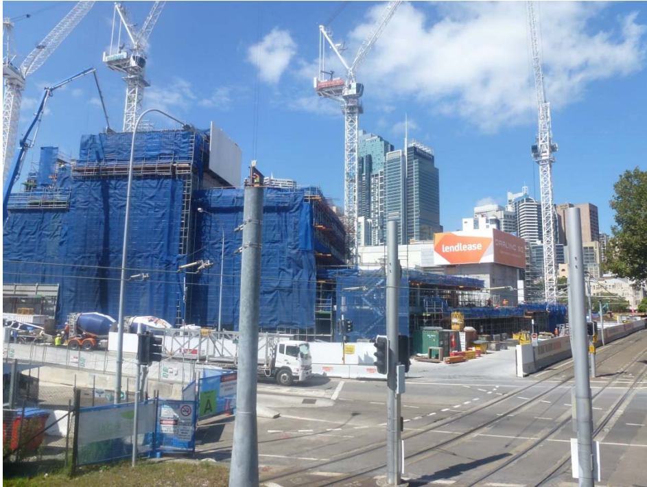
Figure 3 – Construction underway at Darling Square
