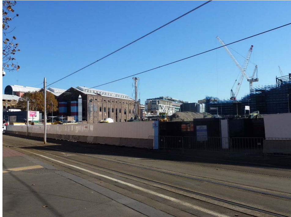
Figure 3 – Construction underway at Darling Square
