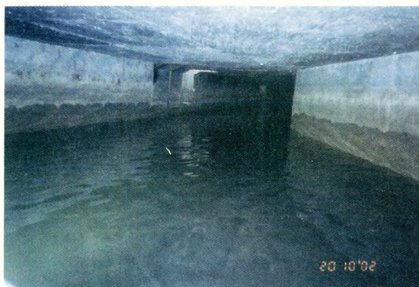
8. DC30A2-CP11 to CP14 (Ch 215.0) Transition & increased water depth
