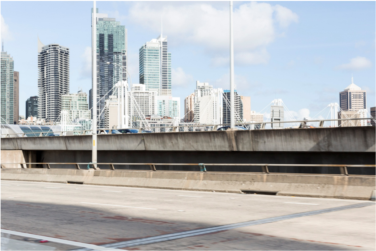
SICEEP Ground View Corridor 8 Existing
