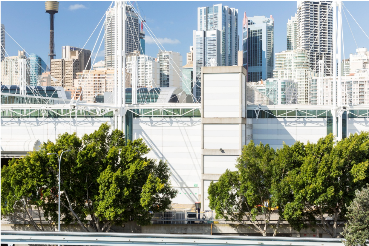
SICEEP Ground View Corridor 14 Existing
