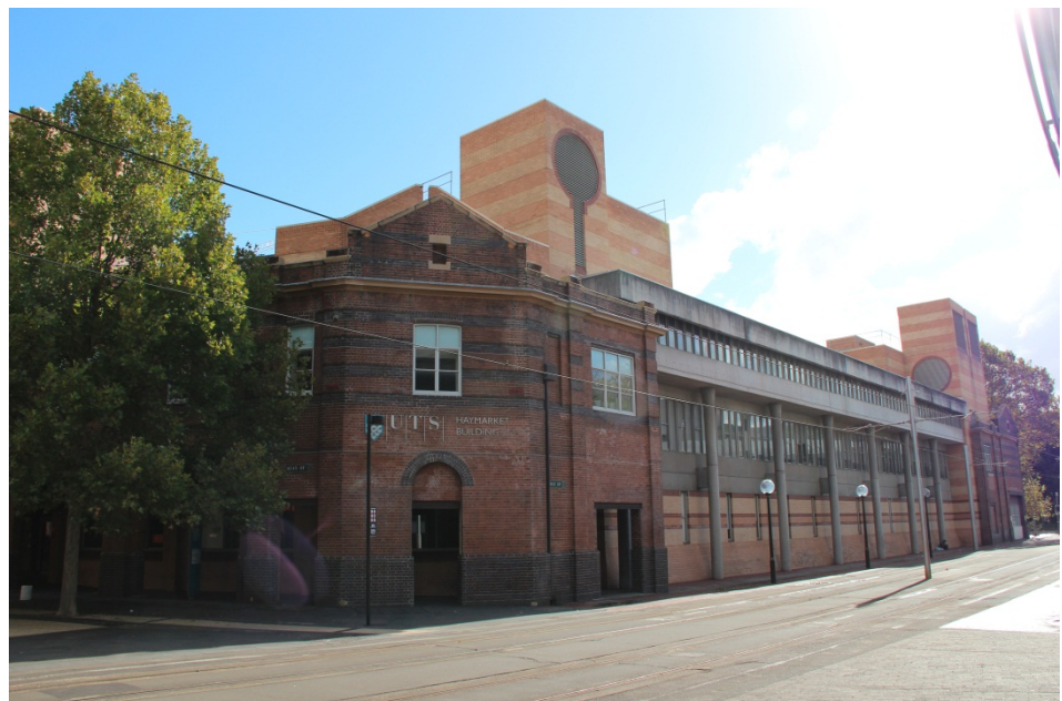
Figure 35 – UTS Haymarket Building 5, viewed from the SEC
