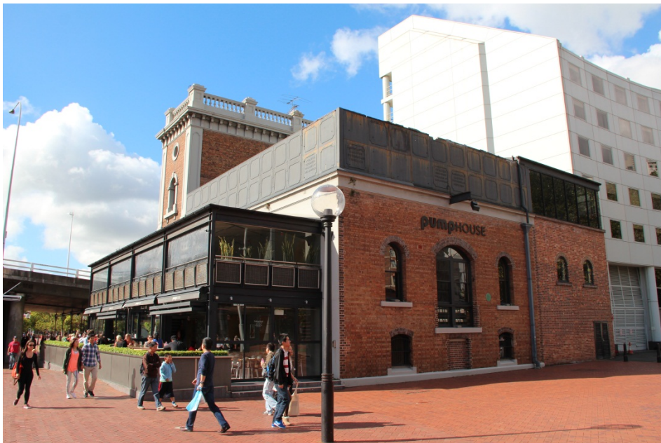
Figure 26 – The Pump house, viewed from the SEC northern forecourt
