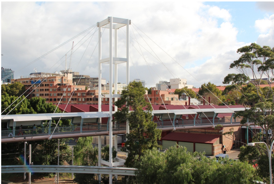
Figure 37 – Former Ultimo Tram Shed with footbridge in the foreground
