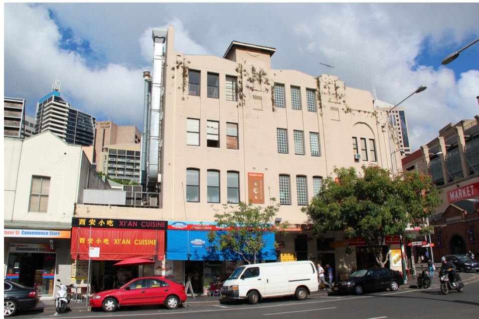
Figure 31 – 90 Hay Street, viewed from the SEC
