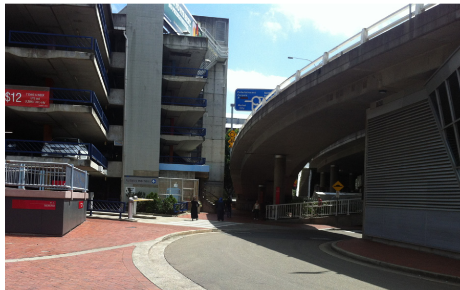
View towards the multi storey SEC car park entry adjacent to Pier Street overpass. Source - HASSELL
