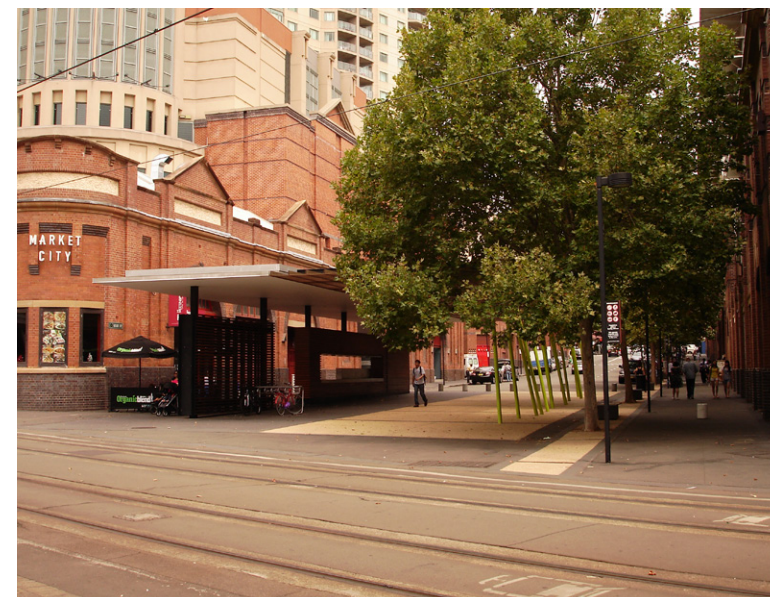
View looking south along Quay Street shelter between the UTS campus and Market City. Source - HASSELL
