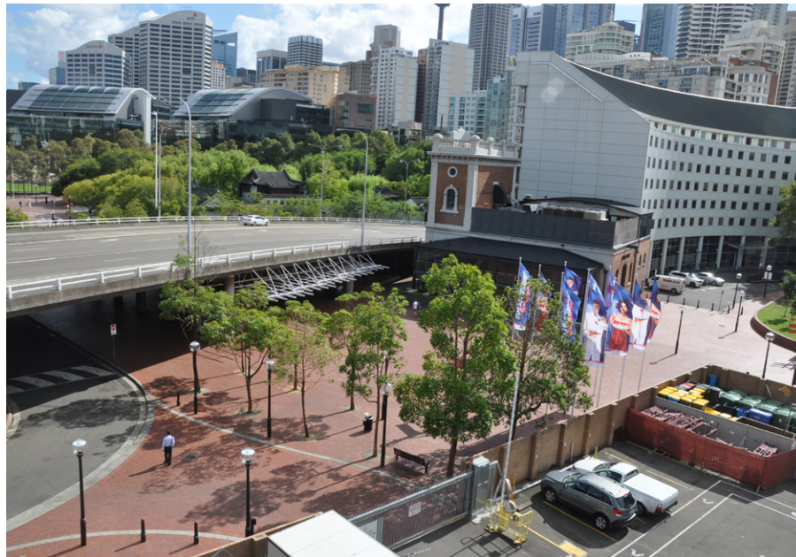
View looking north east from the multi storey SEC car park toward Pier Street overpass with the Pumphouse and paved forecourt below. Source - HASSELL
