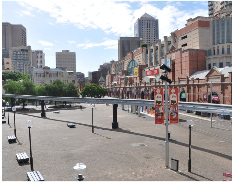
View looking east towards Paddys Markets with existing monorail in foreground. Source - HASSELL
