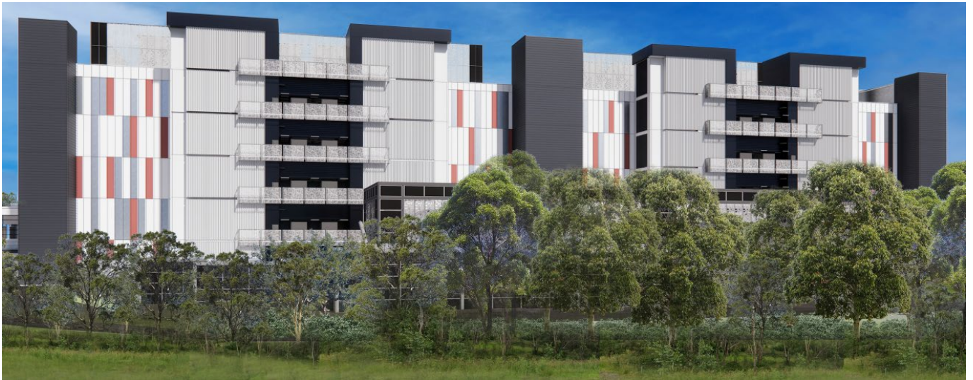
Figure 13 | Original building façade design, viewed from the Great Western Highway
