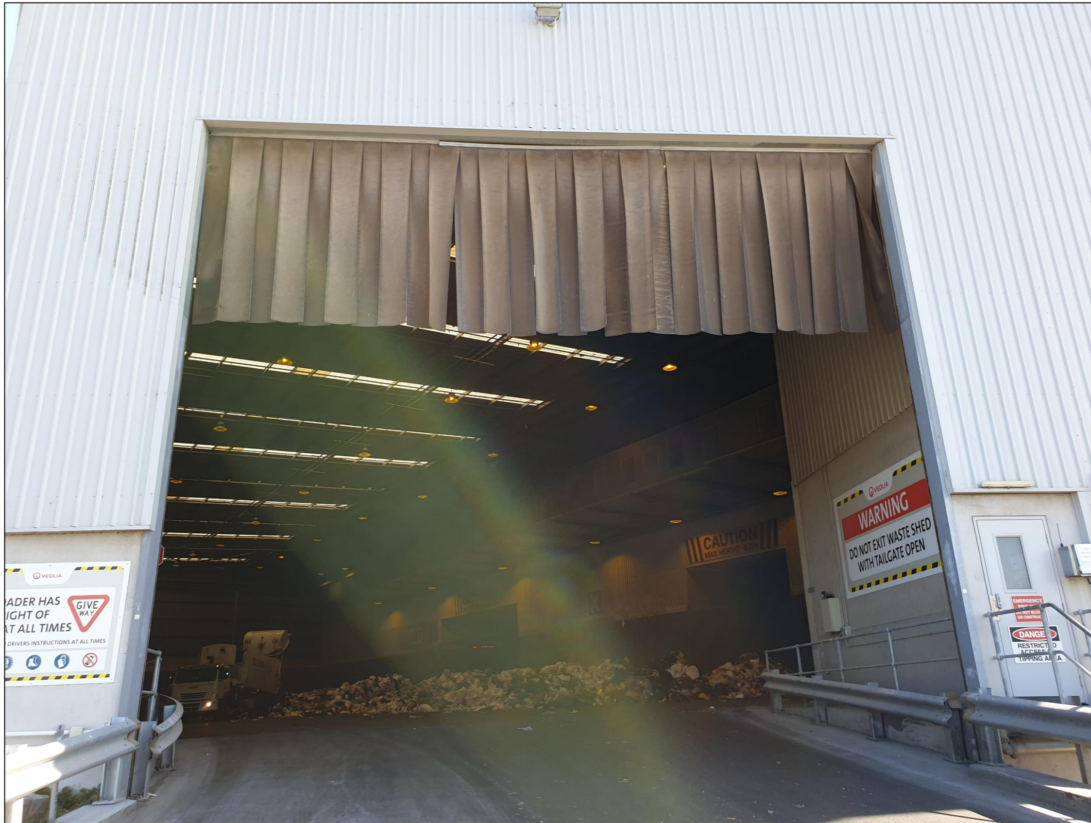
Photo 6 – A picture of the BTT Facility truck entry point as found on 2 October 2019. Note: The truck entrance plastics strips were found to be in good condition
