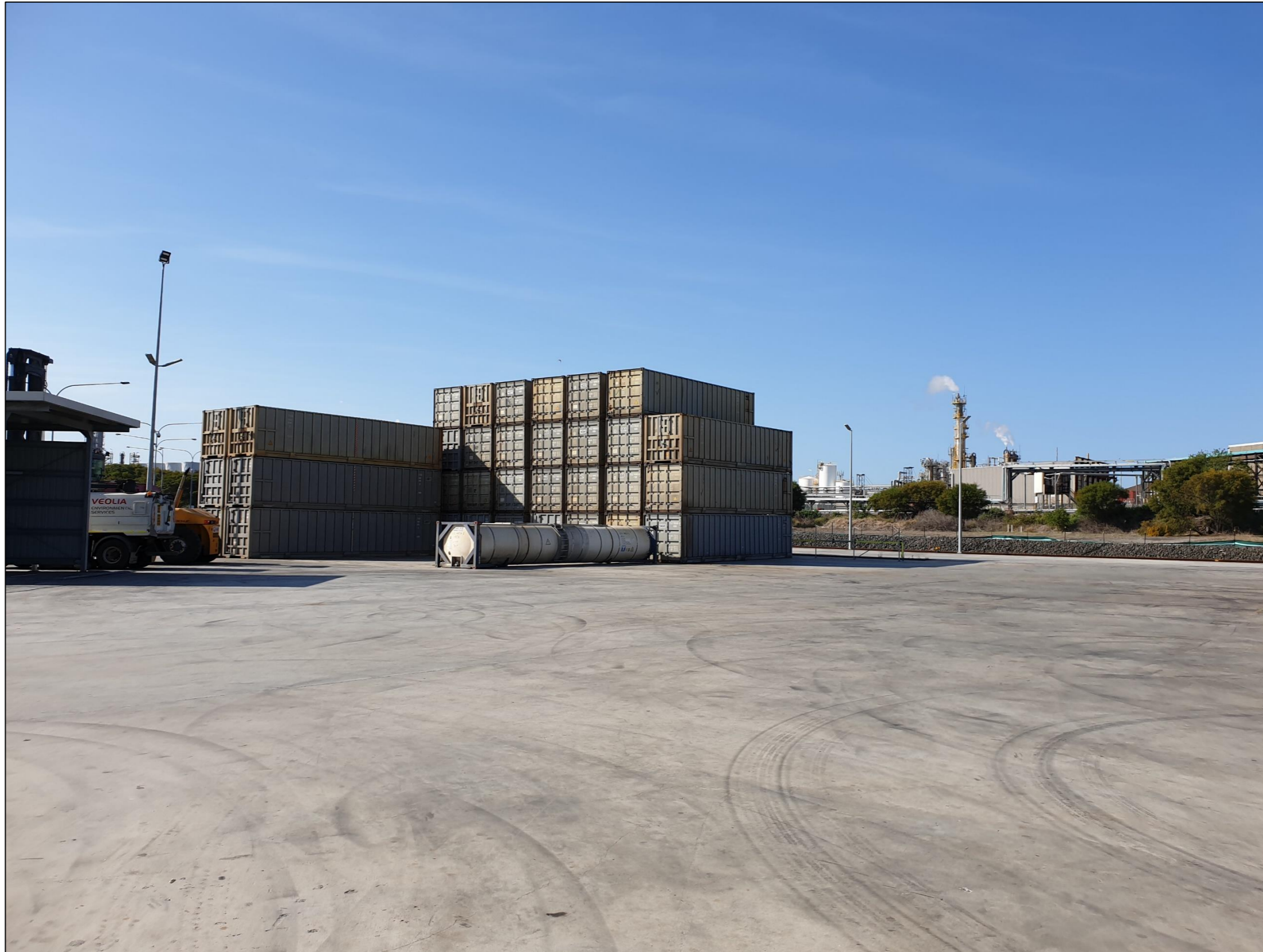
Photo 5 – A picture of the BTT Facility concrete pad facing north-east on 2 October 2019 at 1507 hrs
