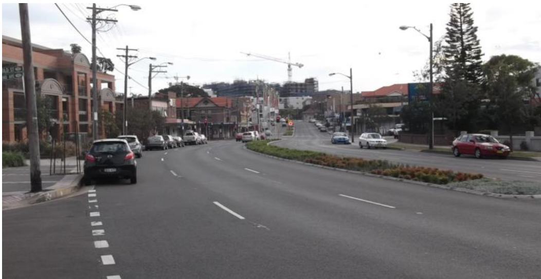
Figure 7 Looking northbound on Bunnerong Road towards Franklin Street and the Matraville Chamber of Commerce (beyond).
