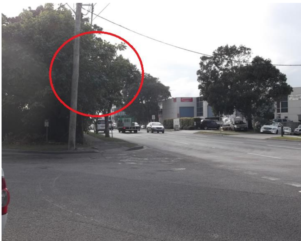
Figure 34 Poor entering sight distance from the McPherson Street approach to Beauchamp Road traffic from the north.
