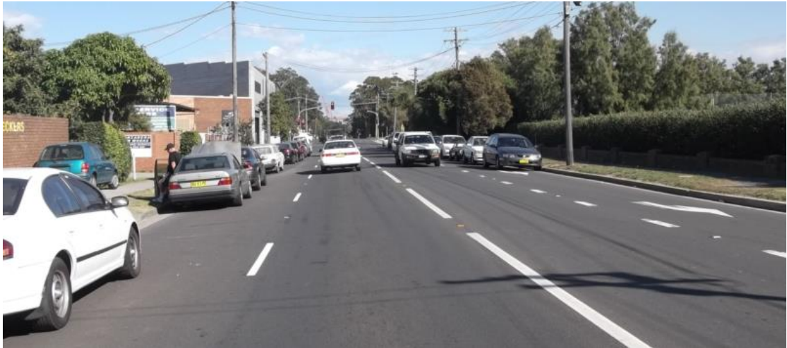
Figure 3 Looking south-west along Beauchamp Road towards Perry Street.
