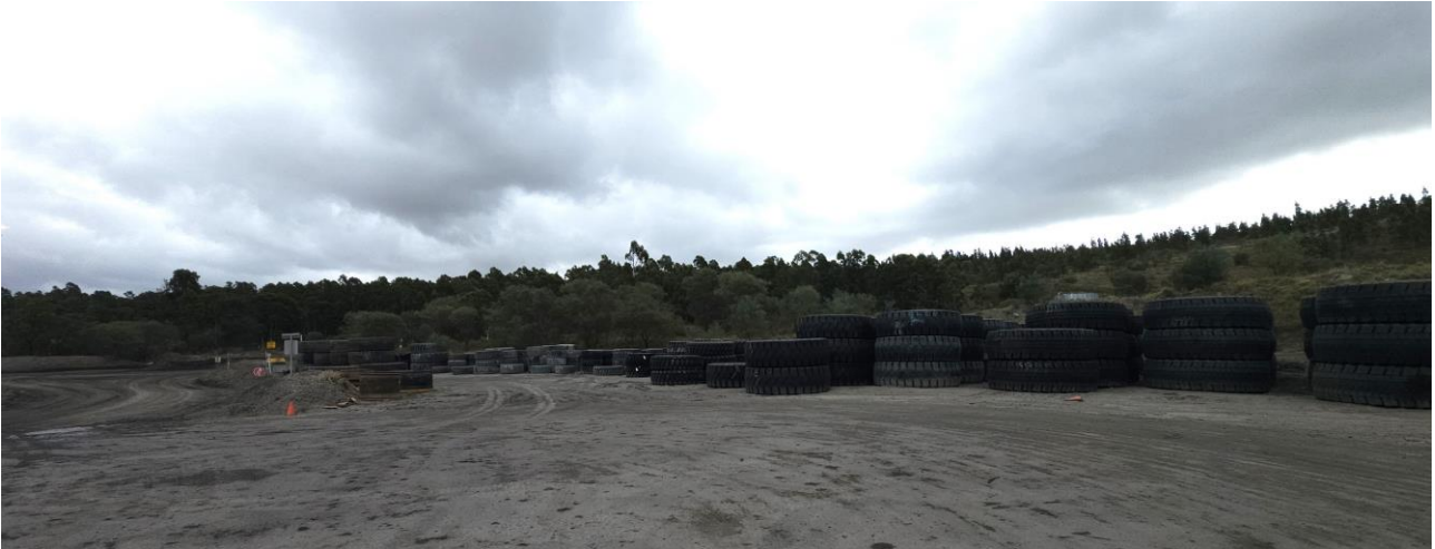
Image 8: Coal Handling Preparation Plant (CHPP) Raw Water Dam
