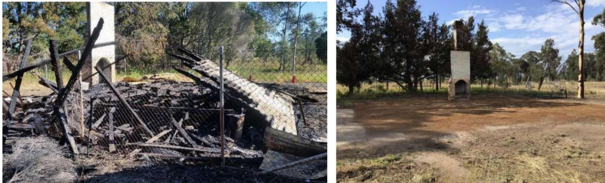
Figure 5-3 – Hebden Public School site following arson event clean up
