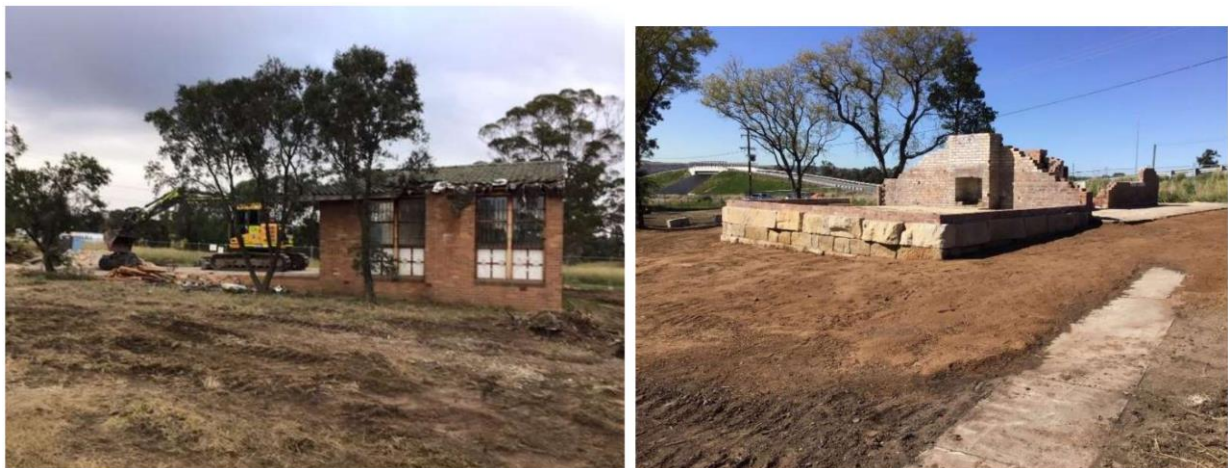
Figure 5-2 – Ravensworth Public School site following arson event clean up
