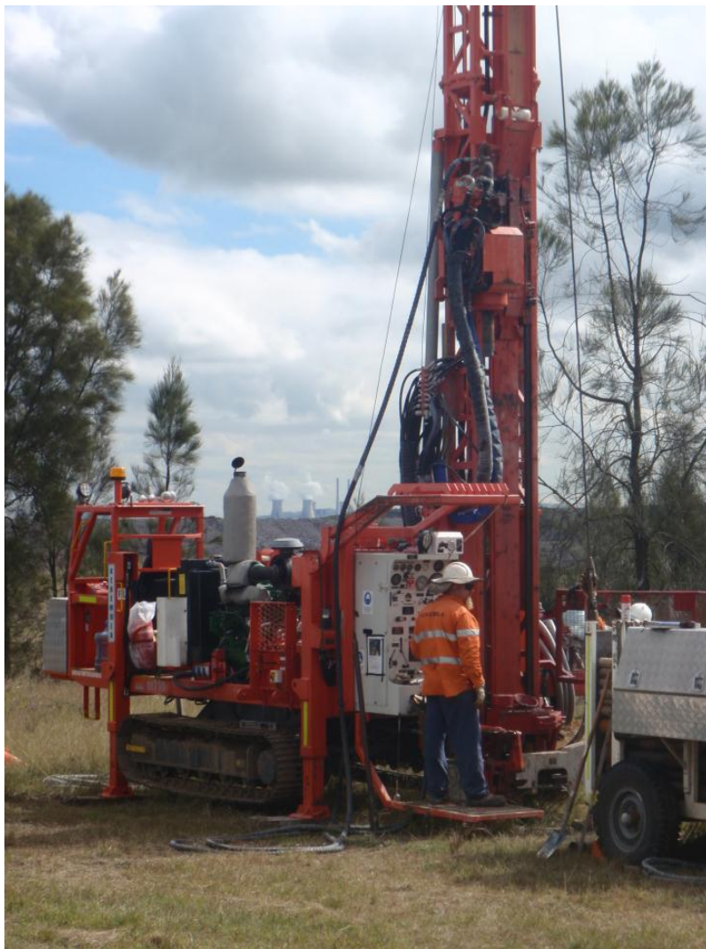
Plate 4 – Installing vibrating wire piezometers south of North Pit
