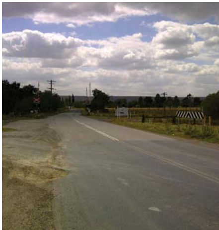
Existing level crossing - Hebden Road.
