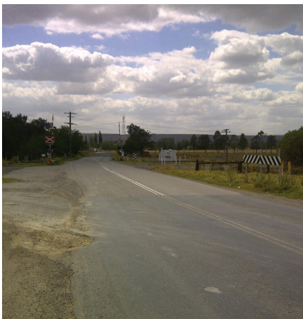
Existing level crossing - Hebden Road.
