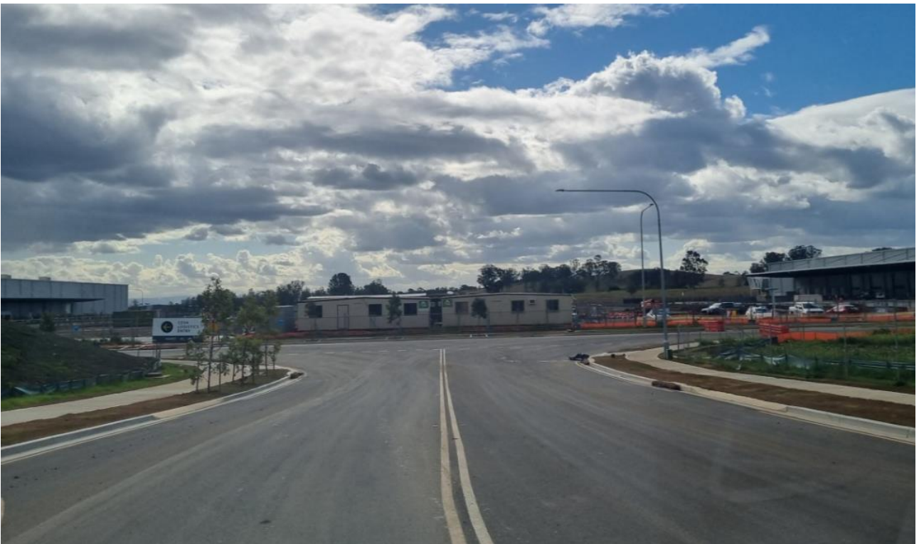
Figure 5: Access Road 4 (looking north towards Access Road 1)
