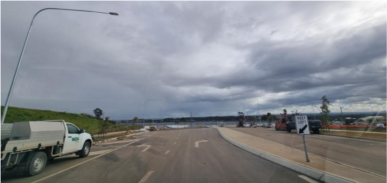
Figure 6: Access Road 1 (looking west towards Mamre Road)
