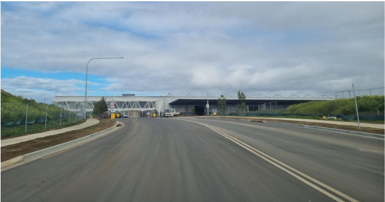
Figure 7: Access Road 4 (looking south)
