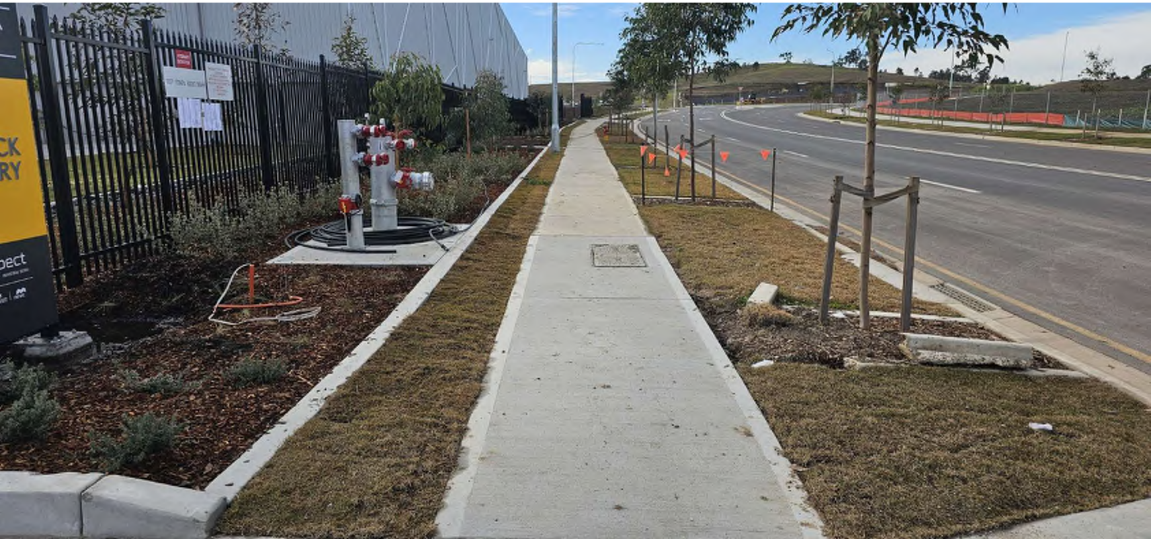
Finished Lot 3 footpath with nature strip grass laid and trees. Broken concrete garden bed by WEM.
