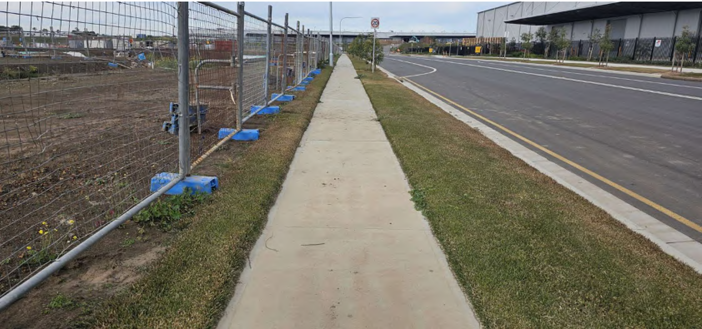
Finished footpath with nature strip grass laid and speed limit sign.
