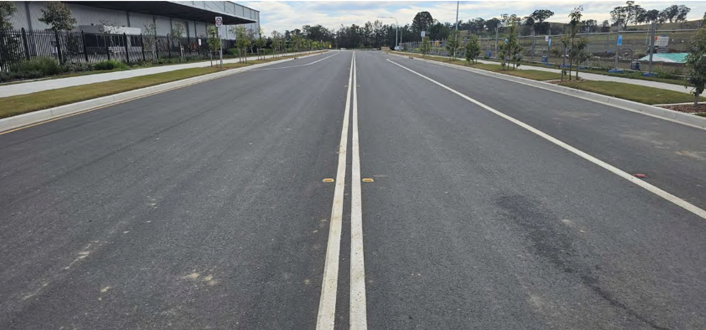
Finished road with asphalt, linemarking, kerbing and signage. Dirt and tyre marks present on the road. Nature strip grass laid and trees installed.
