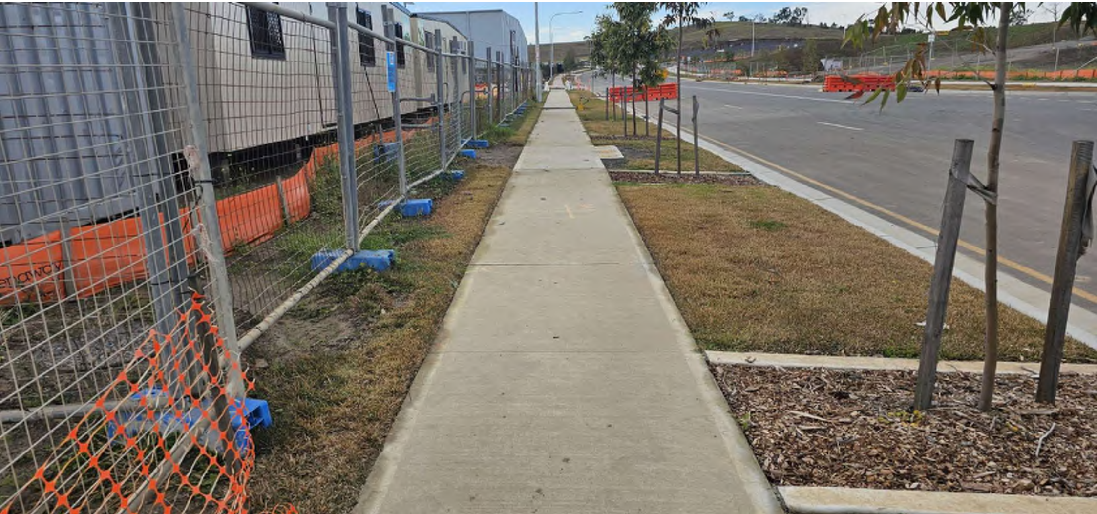
Finished footpath with nature strip grass laid and trees.
