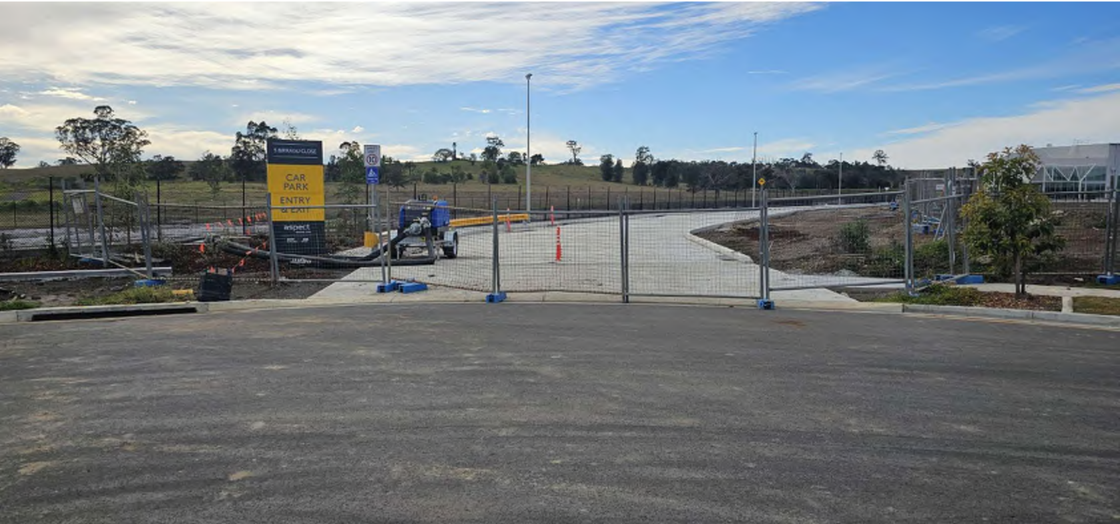
Finished road with asphalt, kerbing and signage. Dirt and tyre marks present on the road. Nature strip grass laid and trees installed.
