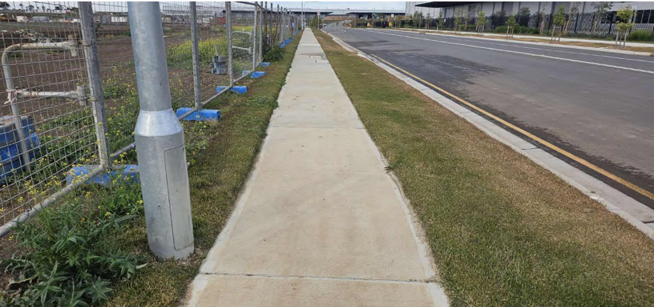
Finished footpath with nature strip grass laid and light post.
