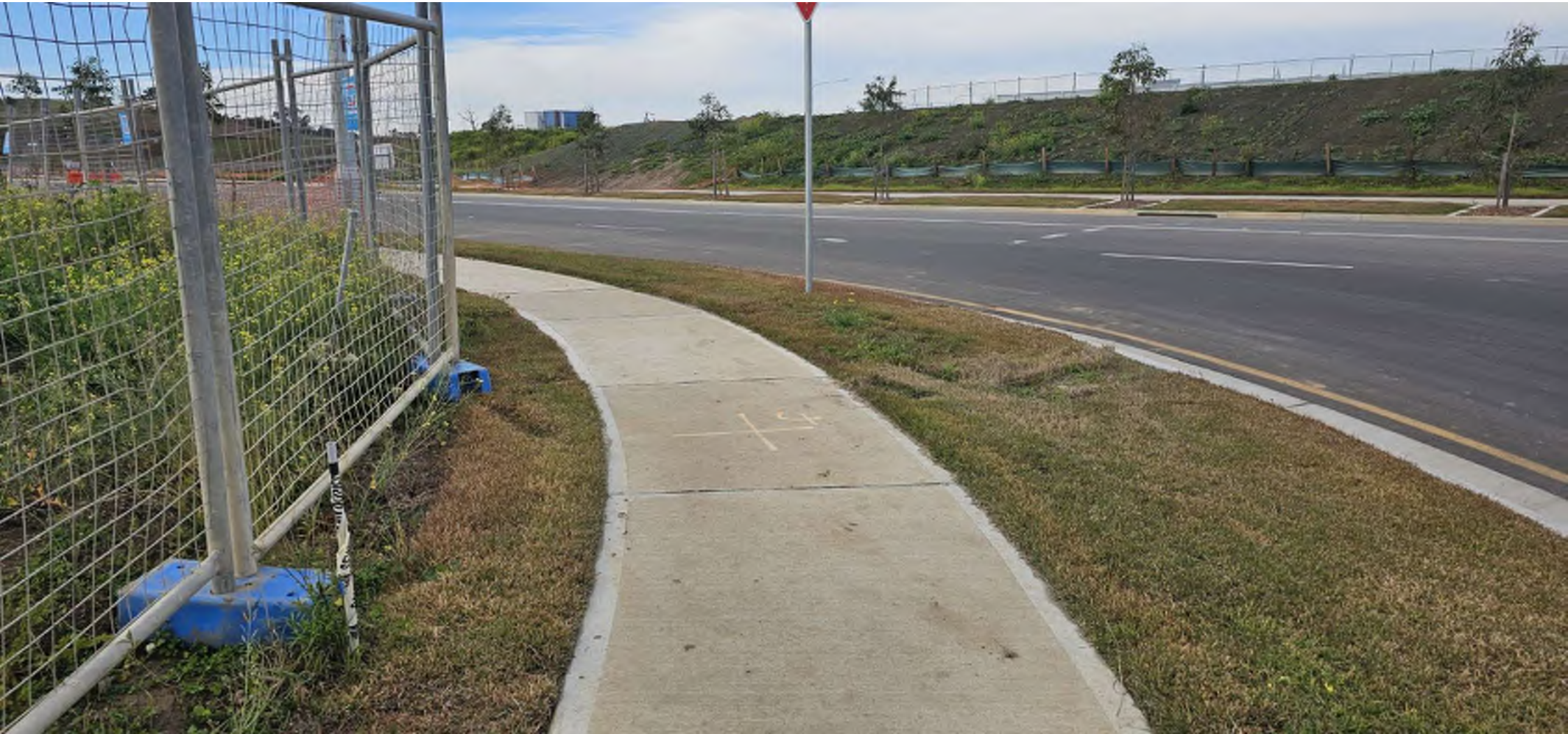
Finished footpath with nature strip grass laid, trees and stop sign.
