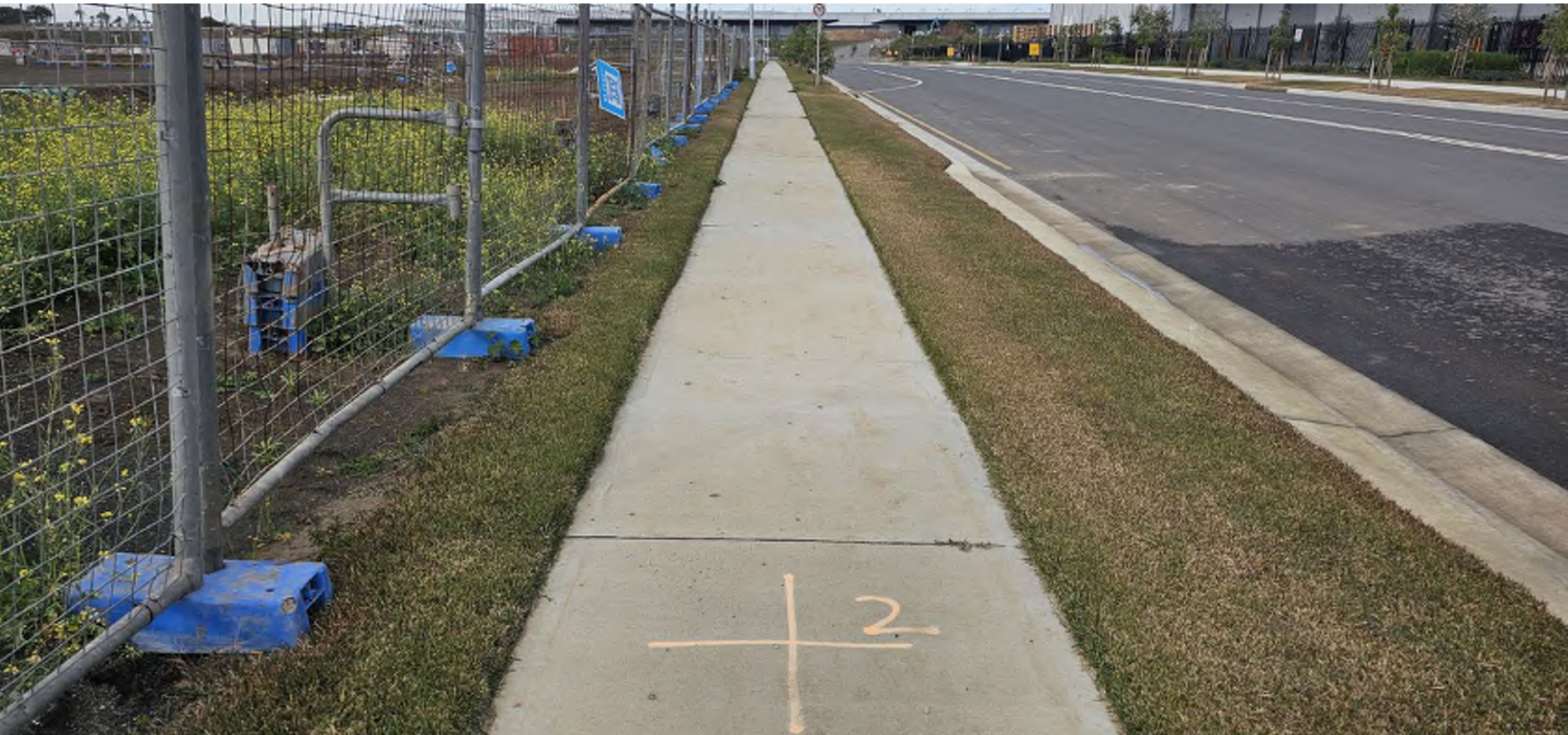
Finished footpath with nature strip grass laid and markings.
