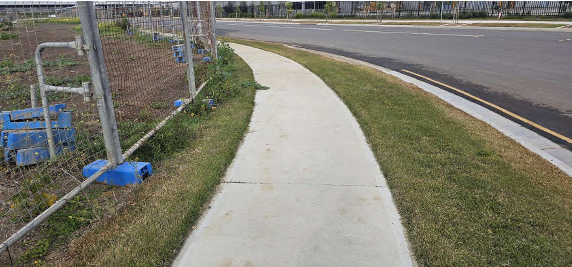
Finished footpath with nature strip grass laid.
