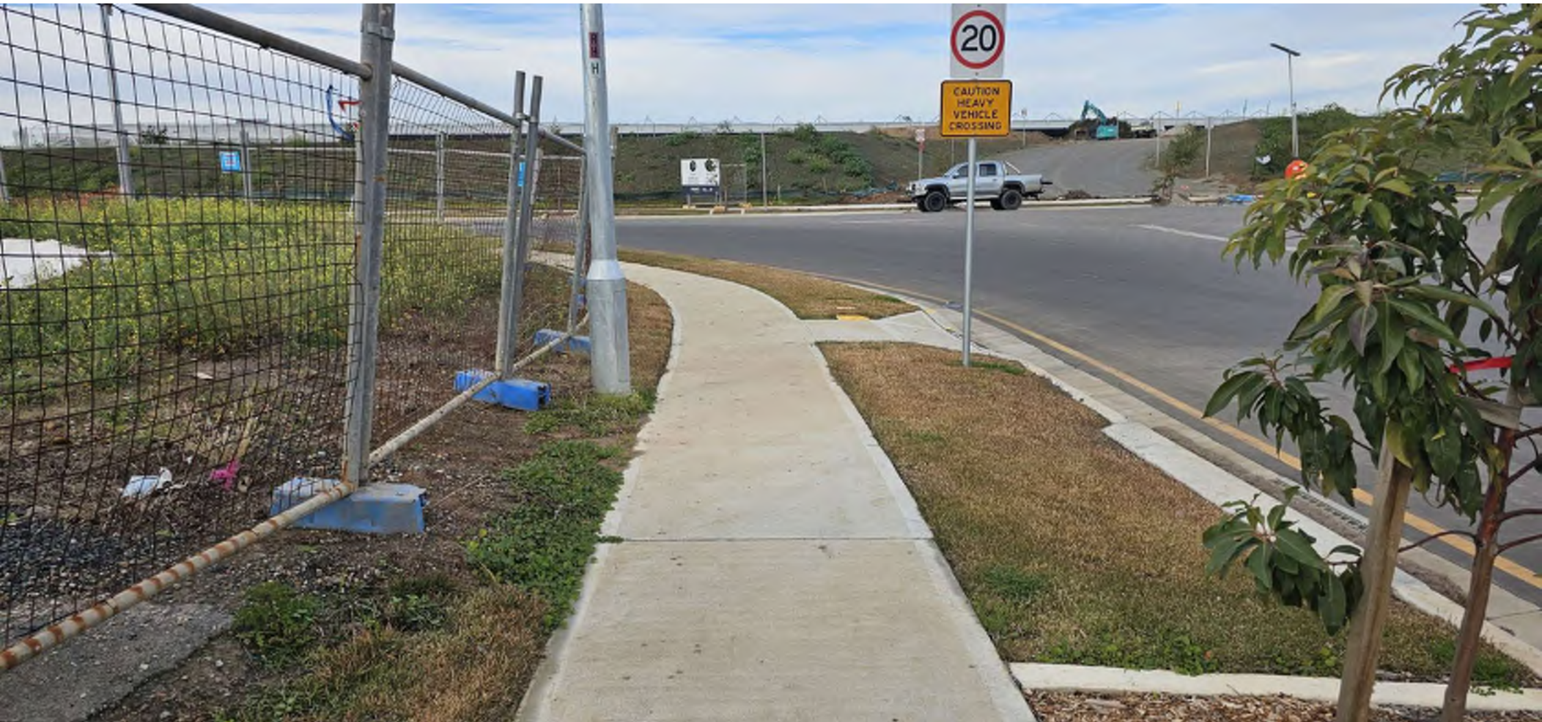
Finished footpath with nature strip grass laid, trees, light post and signage.
