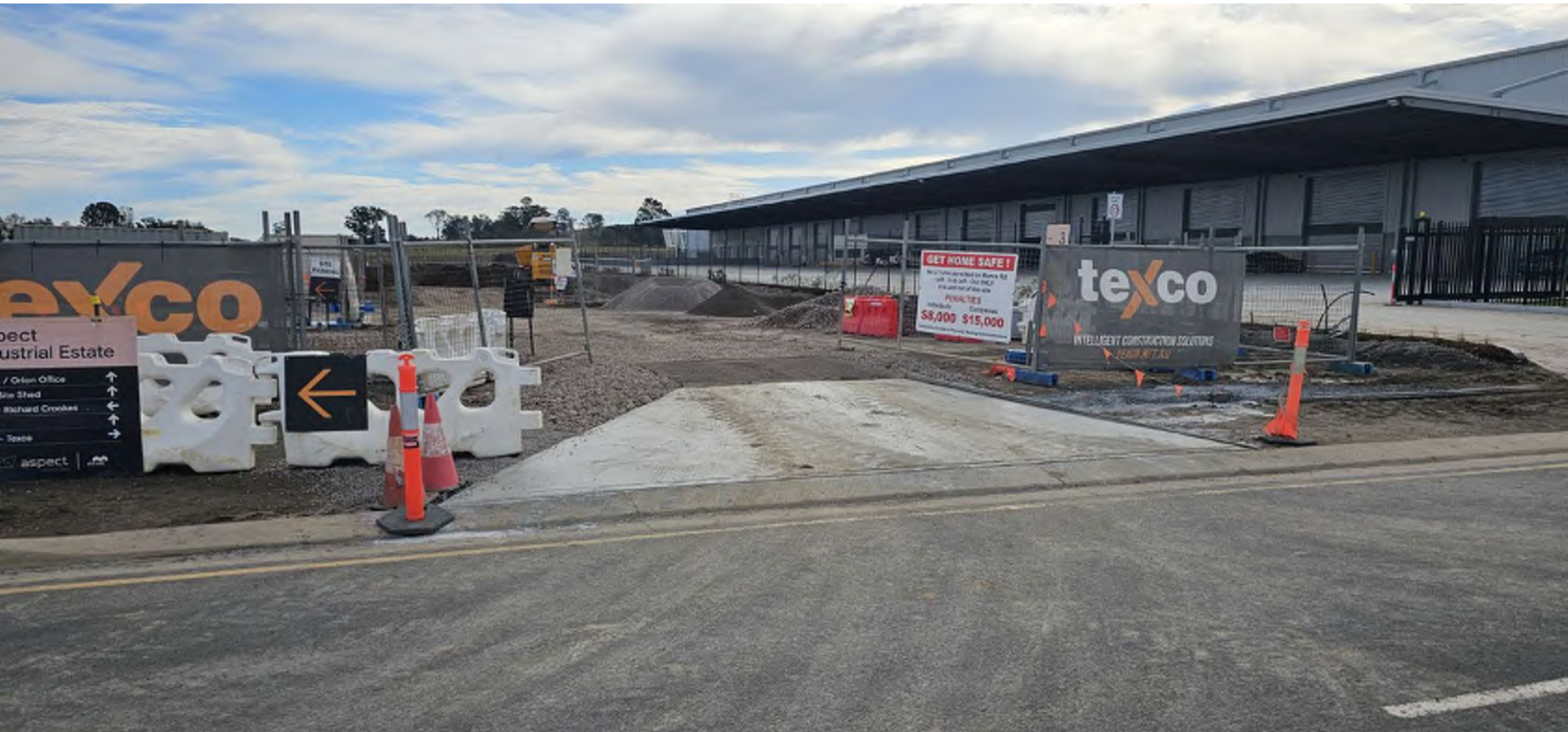
Lot 2 Site Entry. Temporary concrete crossover with cattle grid. Site signage, gate and flagging installed. Lot 2 and Lot 3 adjoining footpath to be poured at Lot 2 completion.
