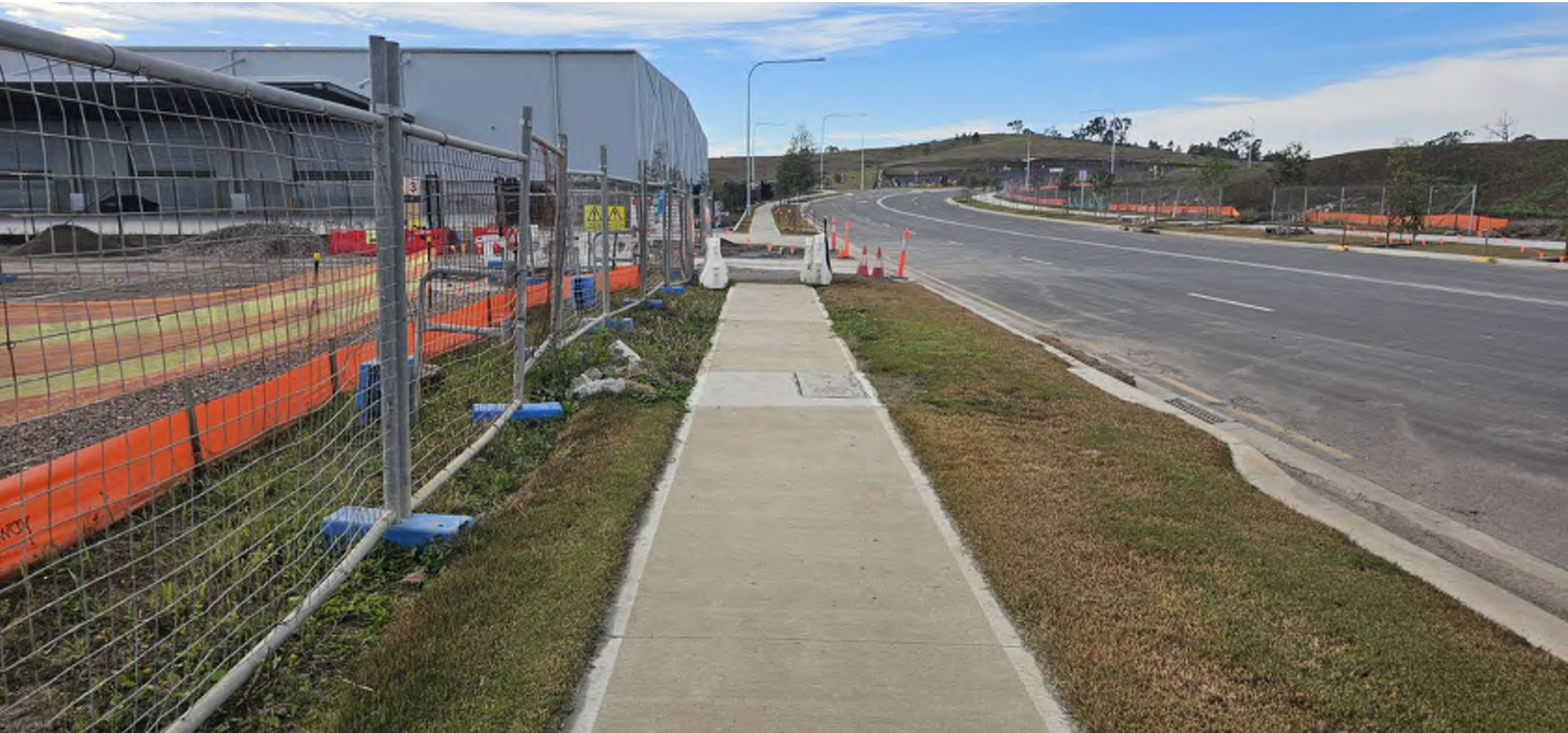
Finished footpath with nature strip grass laid.
