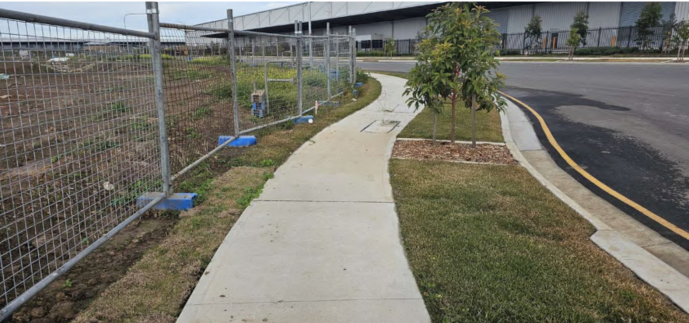
Finished footpath with nature strip grass laid and trees installed.
