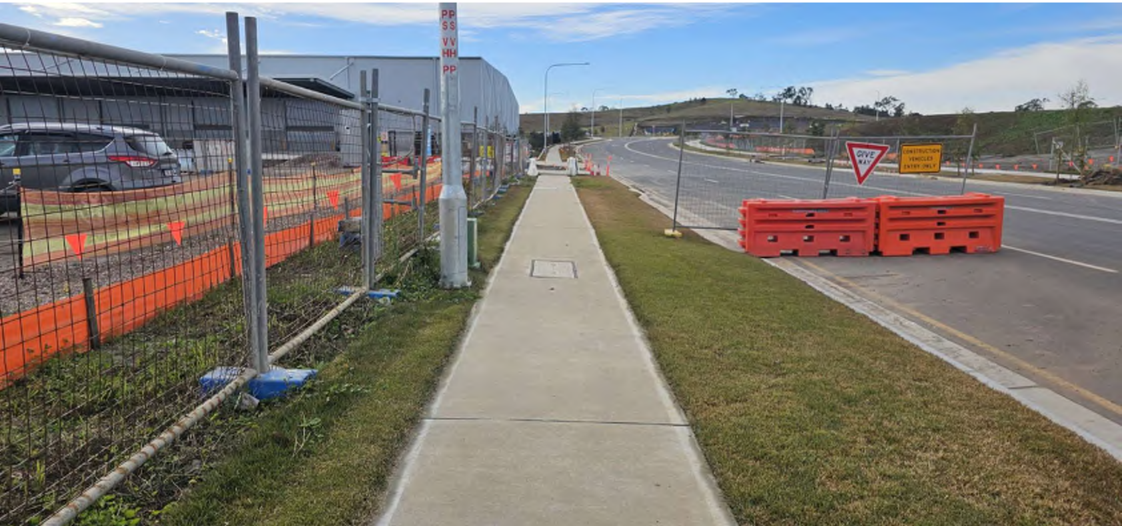
Finished footpath with nature strip grass laid and ligh post.
