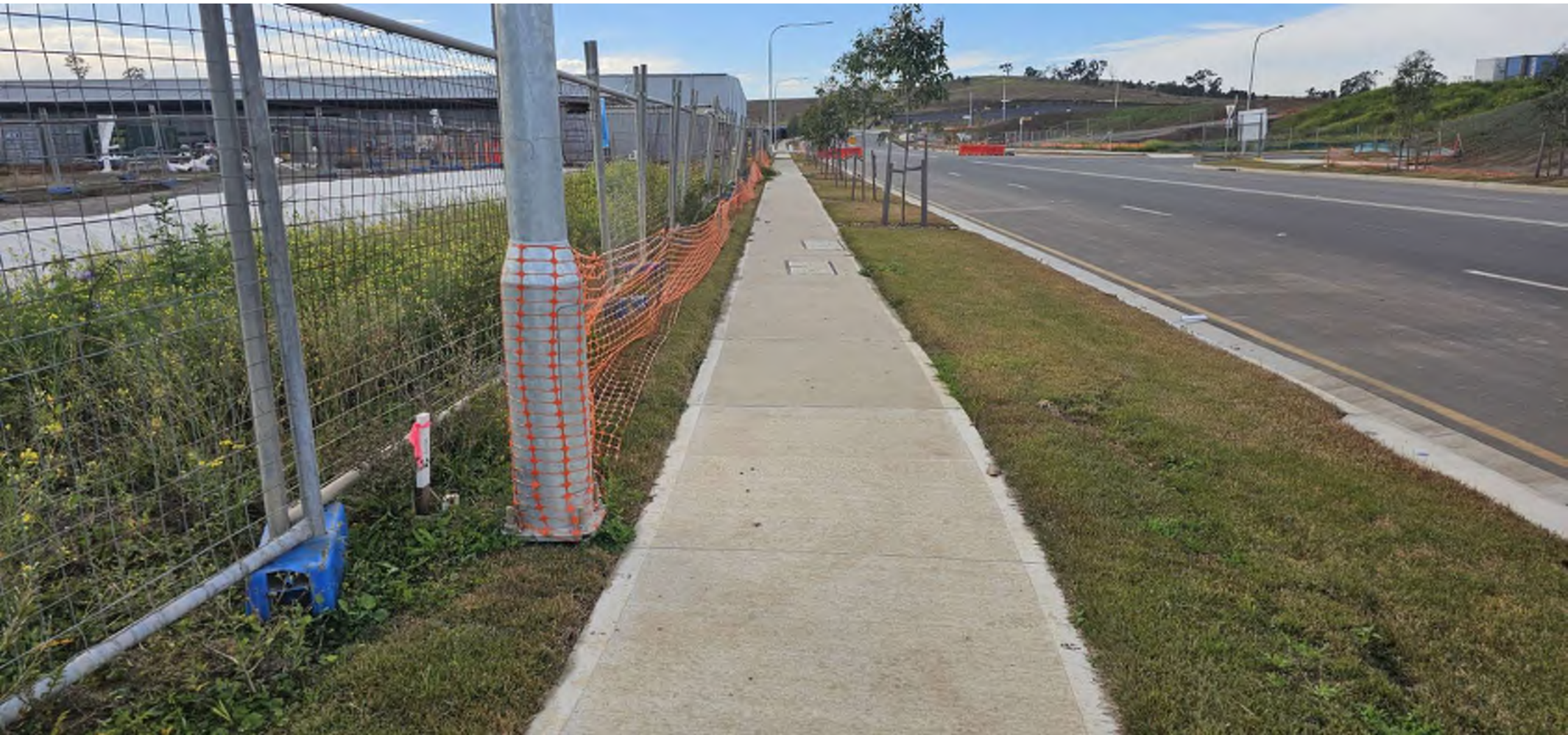
Finished footpath with nature strip grass laid, light post trees.
