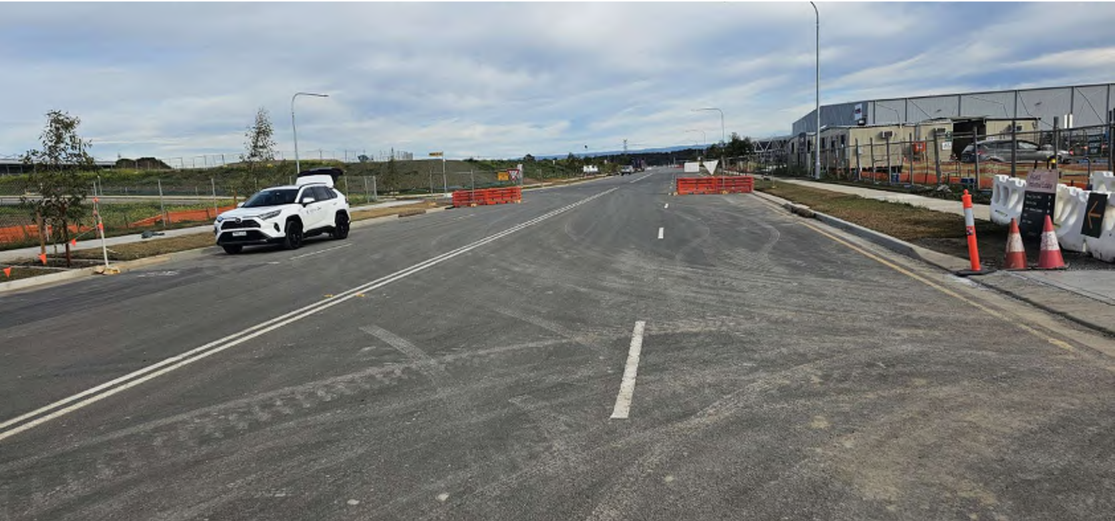
Finished road with asphalt, linemarking and kerbing. Dirt and tyre marks present on the road. Nature strip grass laid and trees installed.
