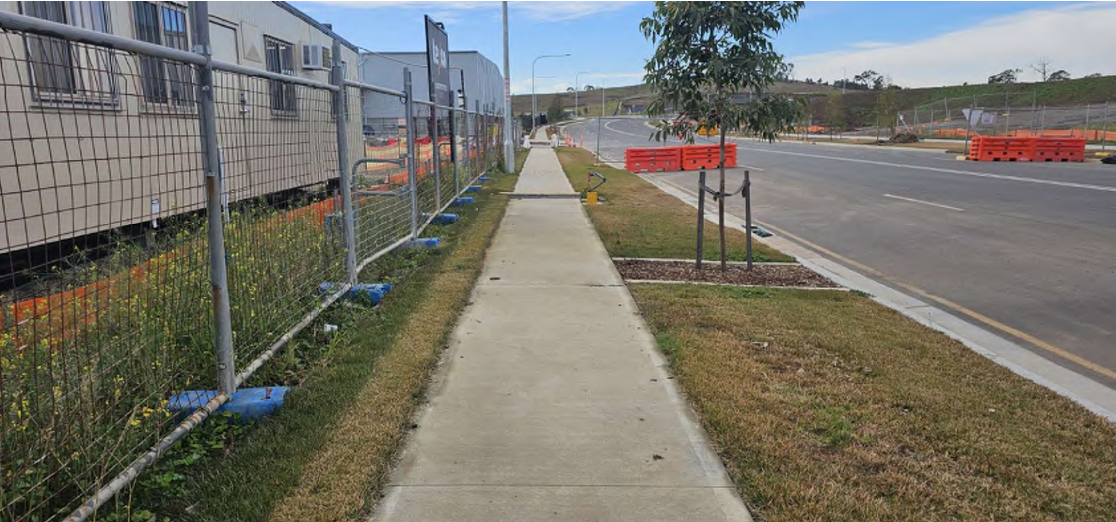
Finished footpath with nature strip grass laid, trees and temporary stand pipe for Lot 2 water supply.
