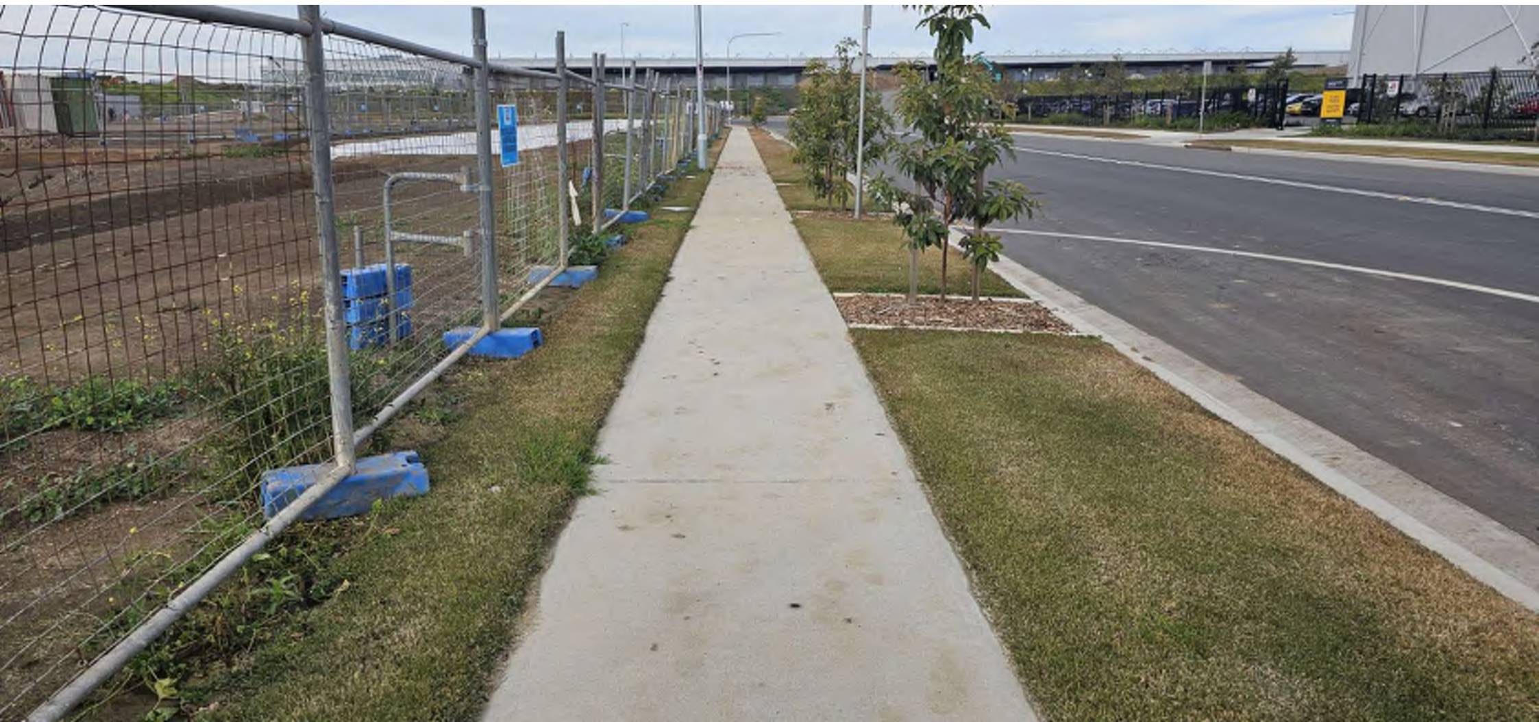
Finished footpath with nature strip grass laid, trees and dirt on footpath and road.
