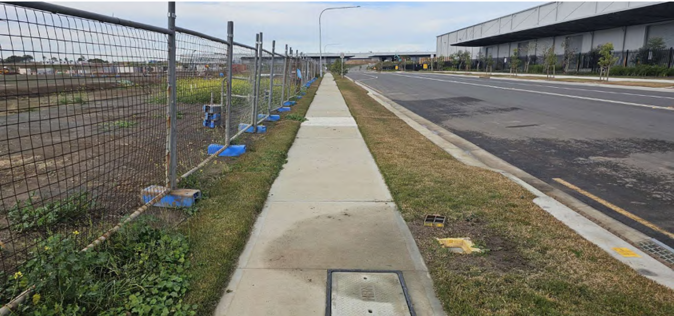
Finished footpath with nature strip grass laid, NBN and stop valve.
