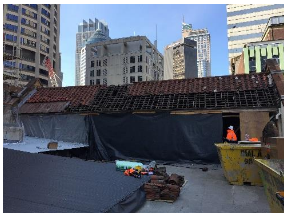
Figure 3 View east to the tiled roof. Tile removal in progress. (Source: GML 2018)
