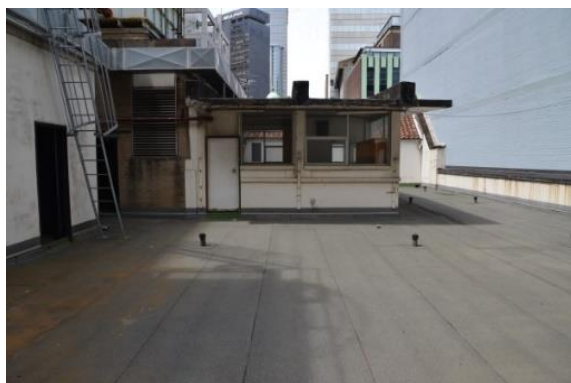
Figure 1 View east towards the main stair structure. (Source: GML 2018)
