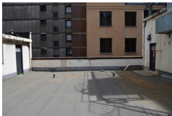
Figure 2 Rooftop looking west to Wynyard Lane. (Source: GML 2018)
