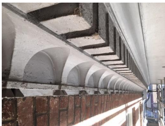
Figure 5 Corbelled cornice which projects over George Street. (Source: GML 2018)
