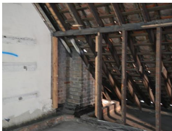
Figure 4 Timber structure of tiled roof (interior view). (Source: GML 2018)
