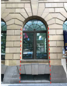
Alterations to the existing condition
