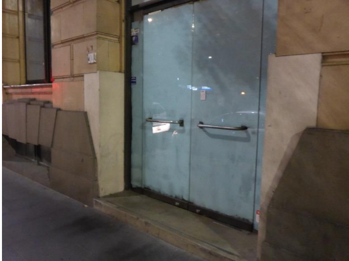
Southern most of the openings in the Carrington Street façade.
