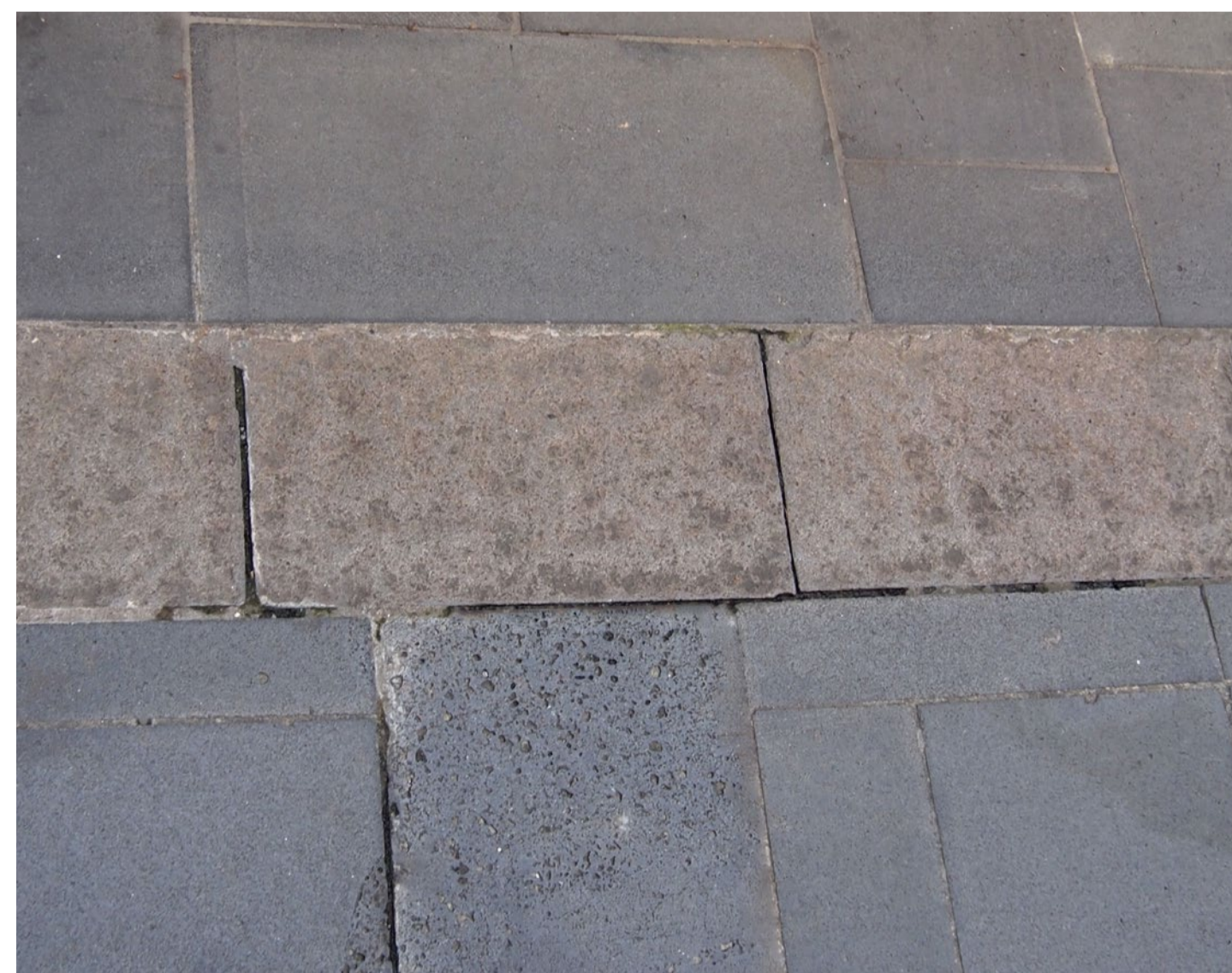
Wynyard Lane - flush (existing) trachyte kerbs
