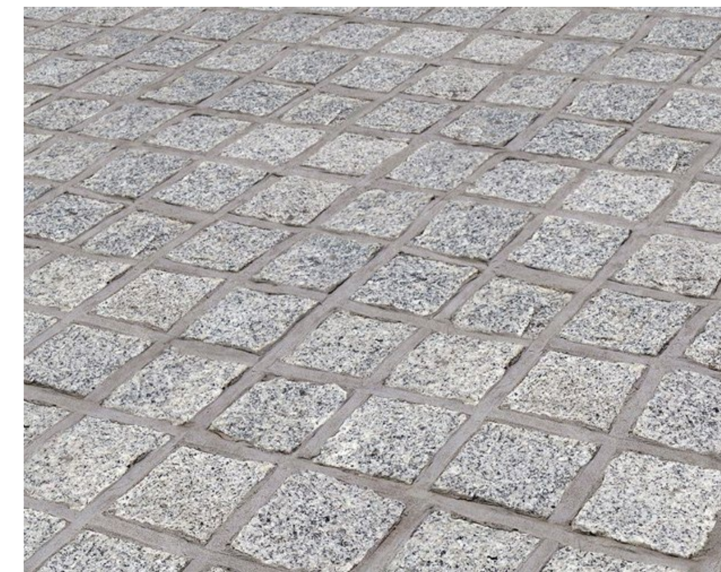
Wynyard Lane - Light grey granite stone setts
