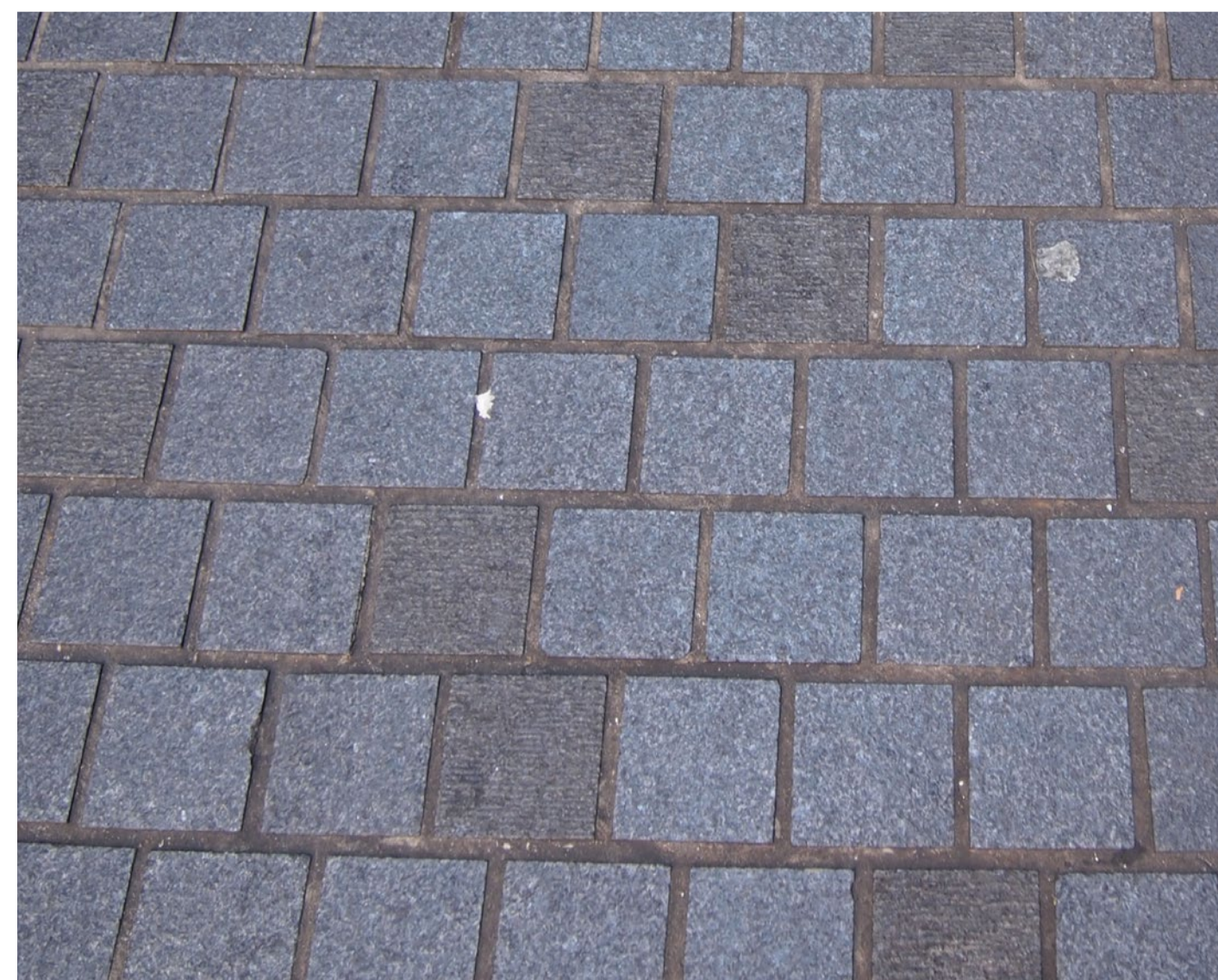
Wynyard Lane - Austral Black granite stone setts
