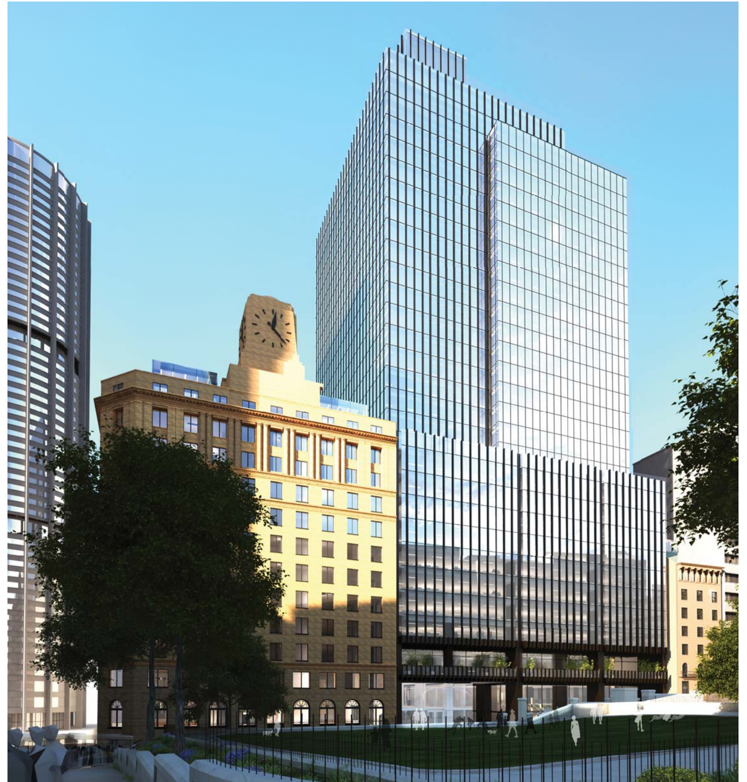
Extract from DA9000 proposed - Illustrative View 01 York and Margaret Street corner view
