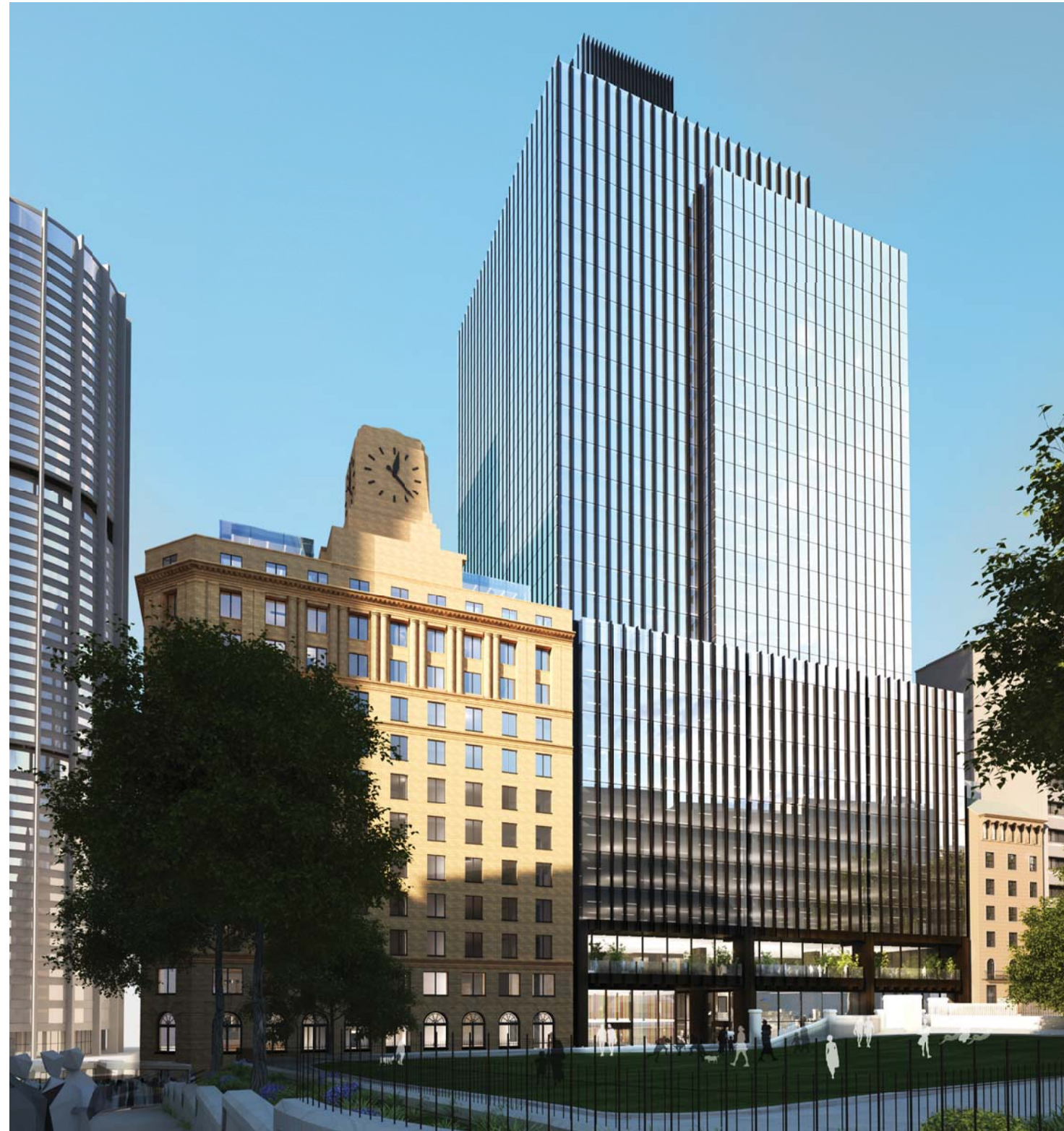
Extract from DA9000 approved - Illustrative View 01 York and Margaret Street corner view
