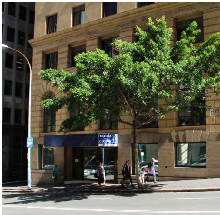
Photo: Margaret Street elevation with existing entrance and canopy
