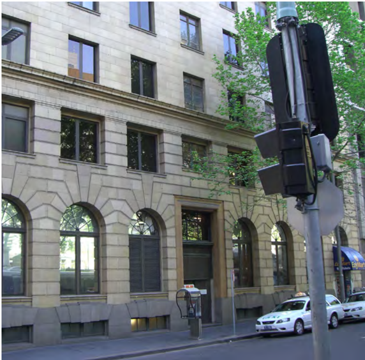
Photo: Carrington Street elevation with original door opening in centre of picture
