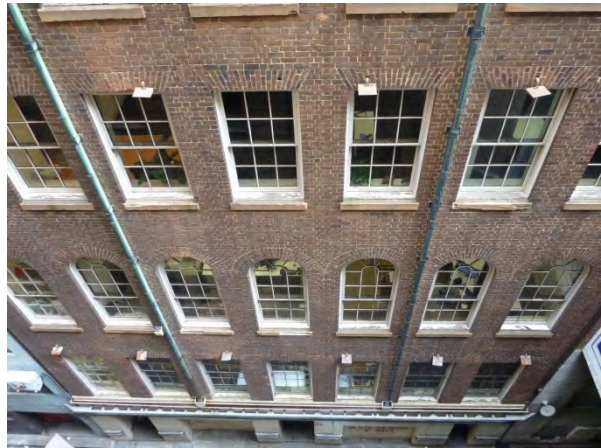
Figure 3.17 View down the Wynyard Lane facade of Beneficial House, showing original windows with sandstone sills. (Source: GML 2014)
