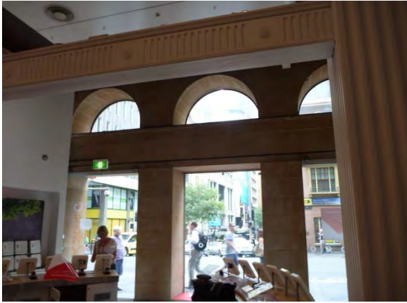
Figure 3.22 Internal fit-out (from c2003), ground floor, looking towards George Street. (Source: GML 2014)
