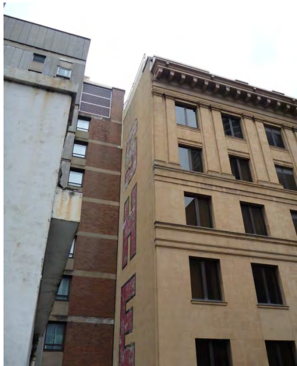
Figure 3.9 Upper part of Wynyard Lane facade of the former Shell House, showing the dentilated cornice and original 'Shell' sign on the southern wall. (Source: GML 2014)
