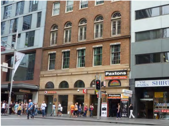
Figure 3.16 George Street facade of Beneficial House, showing the original fanlight windows. (Source: GML 2014)
