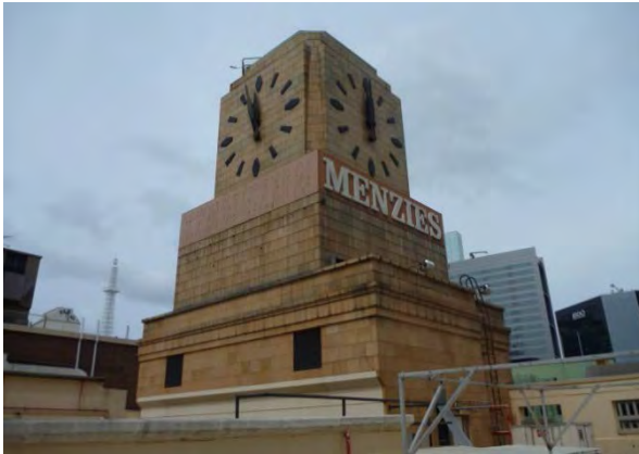
Figure 3.10 Clock tower of the former Shell House, showing the original clock, with glazed terracotta tile cladding and later aluminium signs below. (Source: GML 2014)
