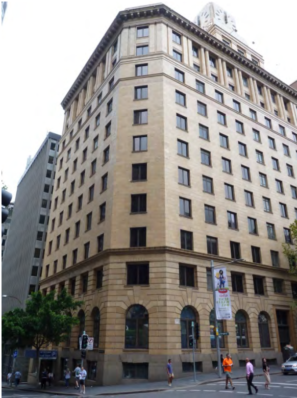
Figure 3.2 Former Shell House, 2–12 Carrington Street. (Source: GML 2014)
