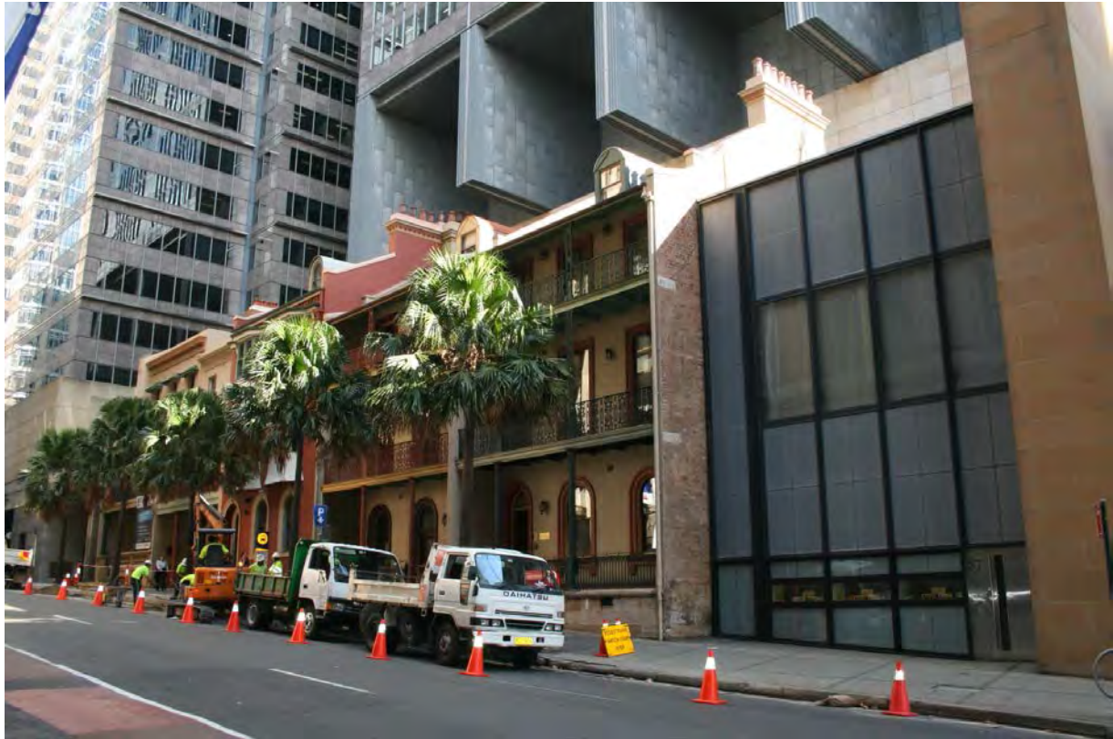
Figure 6.3 Precedent of a cantilever over a heritage item in the City of Sydney LGA—the Governor Phillip tower of the Phillip Street terraces (listed on the State Heritage Register). (Source: GML 2013)
