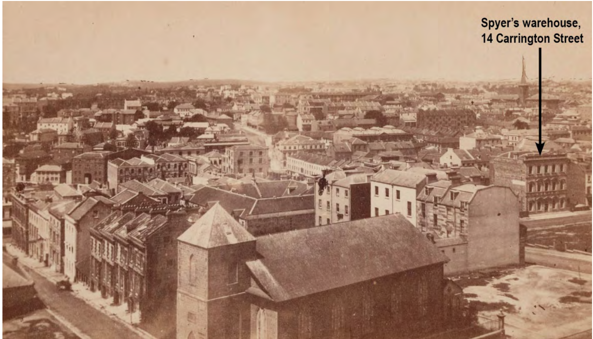
Figure 2.18 1870 view taken from the spire of St Philip's Church looking southeast. Wynyard Park and Spyer's Warehouse at 14 Carrington Street can be seen to the right of the image. (Source: Historic Houses Trust)
