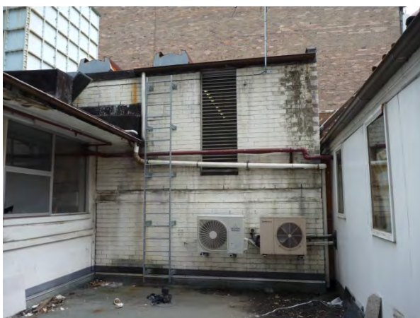
Figure 3.20 Roof of Beneficial House, showing the 1970s store over the light well on the left, original parapet to the right (the later modifications) and services in the centre. (Source: GML 2014)
