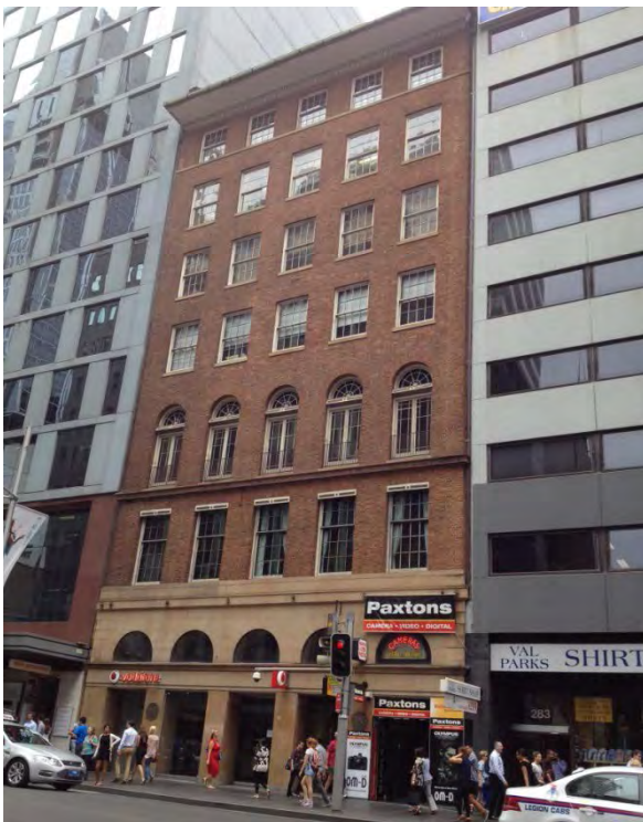
Figure 3.4 Beneficial House, 285–287 George Street. (Source: GML 2014)
