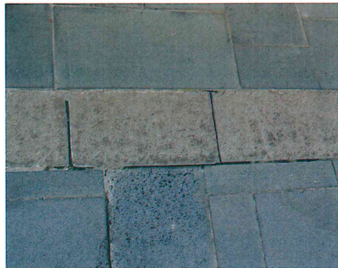
Wynyard Lane - flush (existing) trachyte kerbs
