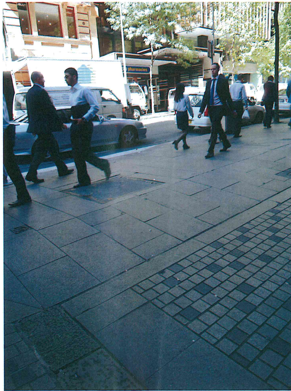
Footpath continuation across across Wynyard Lane entry with vehicle ramp
