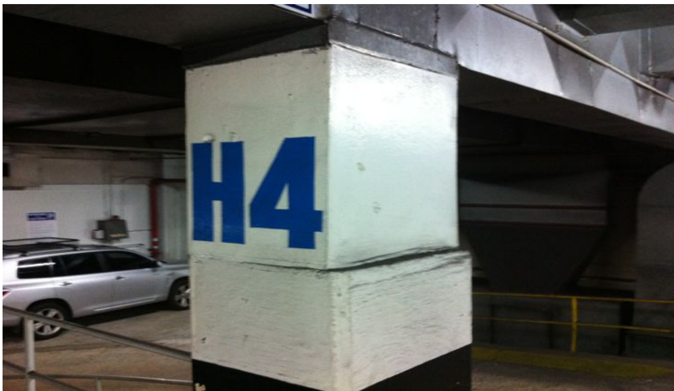
Photo 32: Encapsulated columns containing asbestos lagging insulation located throughout the Upper and Lower Tunnels of the Wynyard Lane Car Park.
