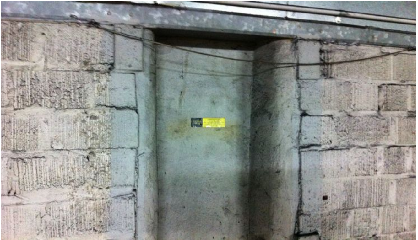
Photo 33: Encapsulated columns containing asbestos lagging insulation located throughout the Upper and Lower Tunnels of the Wynyard Lane Car Park.
