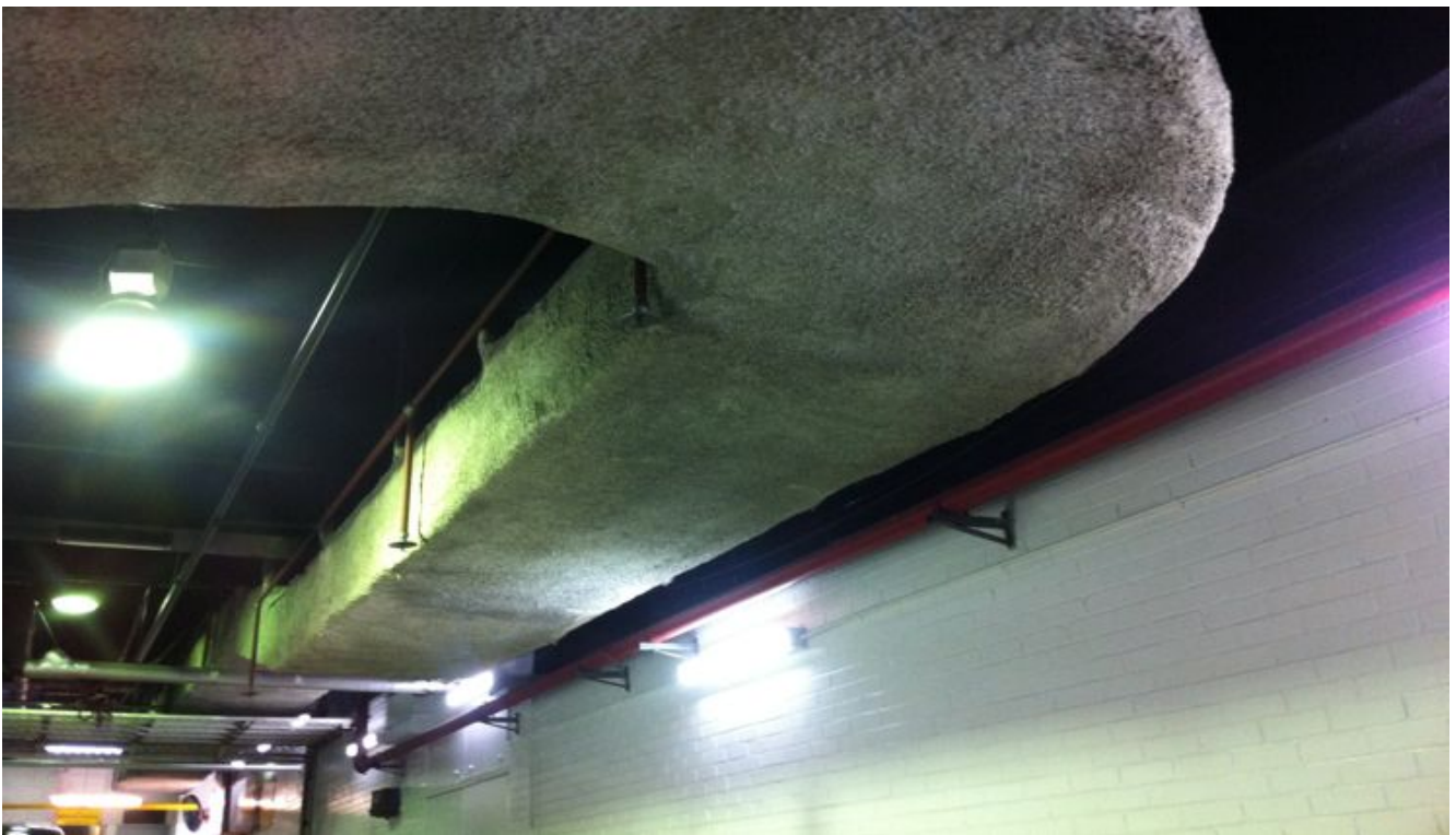
Photo 54: Sprayed SMF insulation located adjacent to the entrance to the Wynyard Lane Car Park.
