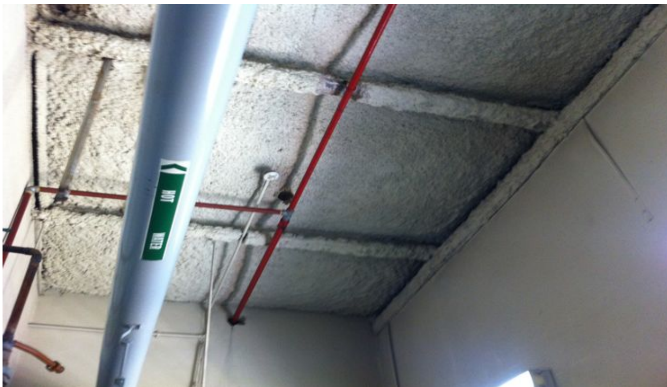
Photo 48: Sprayed SMF insulation on the ceiling of the Boiler Room on the Rooftop Level of the North Wing – Menzies Hotel.
