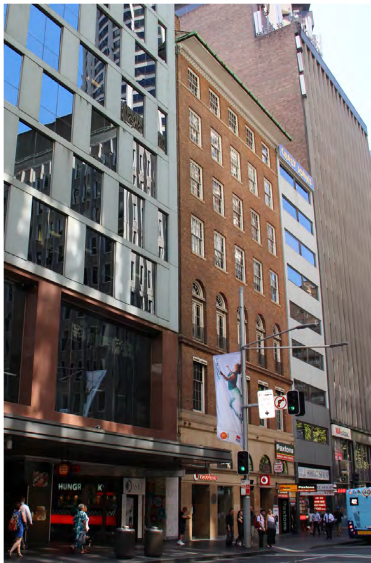
285 George Street, existing condition with awning removed. George Street looking north.
