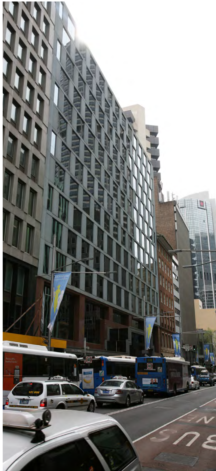
301 George Street and 285 George Street beyond, existing condition.
