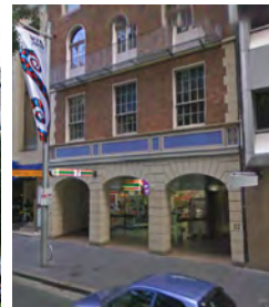
30 Carrington Street • Brick • Mid-rise
