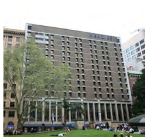
The Menzies, 14 Carrington Street • Brick • Mid-rise
