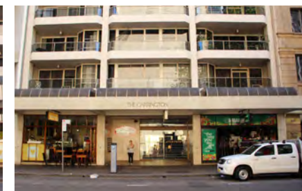
57 - 59 York Street, The Carrington • Concrete • Traditional mid-rise
