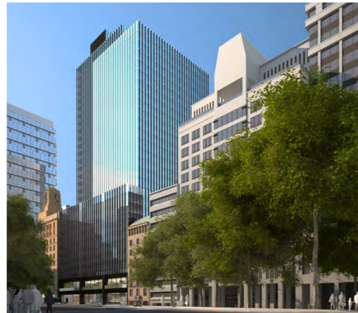
Fig. 1: Looking north-east at York Street and Erskine Street junction
