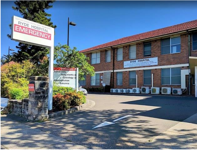
Figure 4 Main Hospital Entrance off Denistone Road
