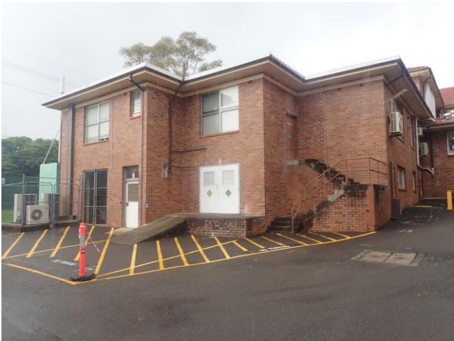
Figure 6 Existing Building on Site
