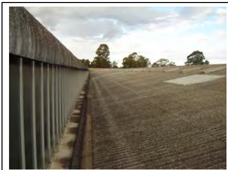
Photograph No.1: An example of an asbestos cement sheet roof
