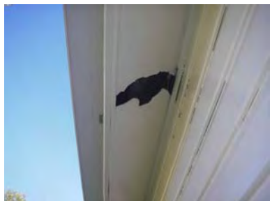
Photo 1. NB8002 Community Health Centre – Eaves
