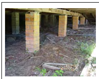
Photo 1. Urunga Community Seaboard Centre – Sub Floor Area
