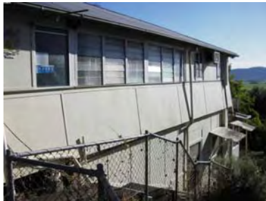
Photo 1. MW05 Cletus Smith Cottage; Exterior – Wall Panels
