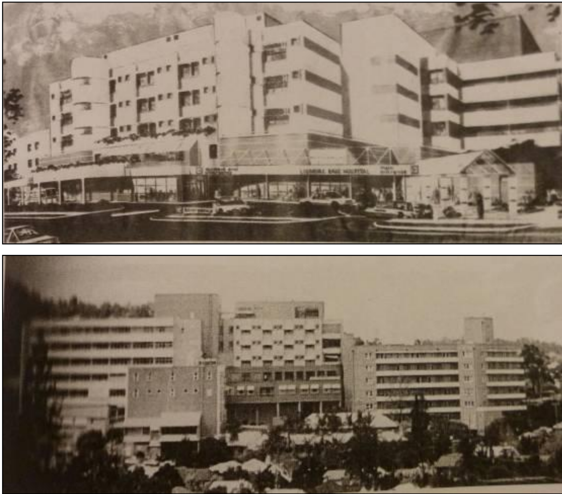
Figure 4.19: The Lismore Base Hospital in 1993 (from Uralba Street) and 2009 (viewed from north)
