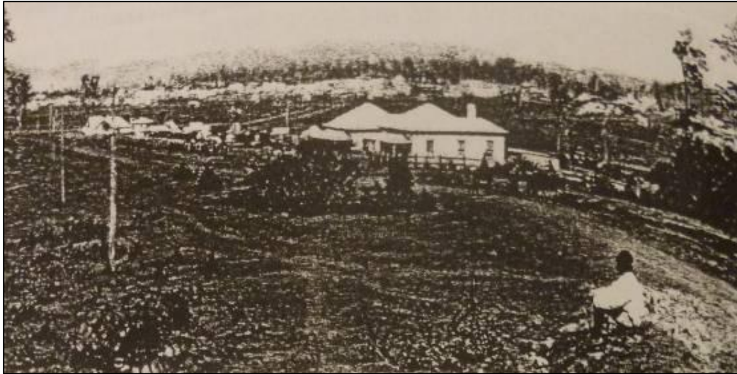
Figure 4.3: View of Lismore looking north-west from Uralba Street below hospital site in 1892
