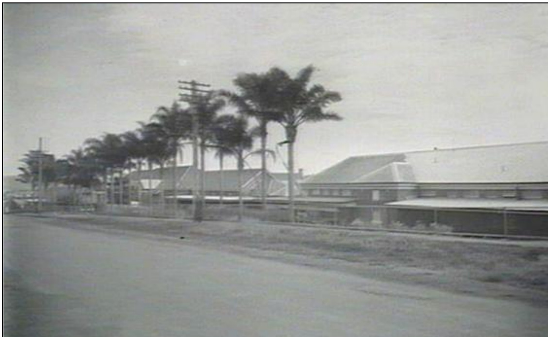
Figure 4.11: Base Hospital, Lismore in August 1936 (Source: State Library of NSW, Government Printing Office 1 - 24314)
