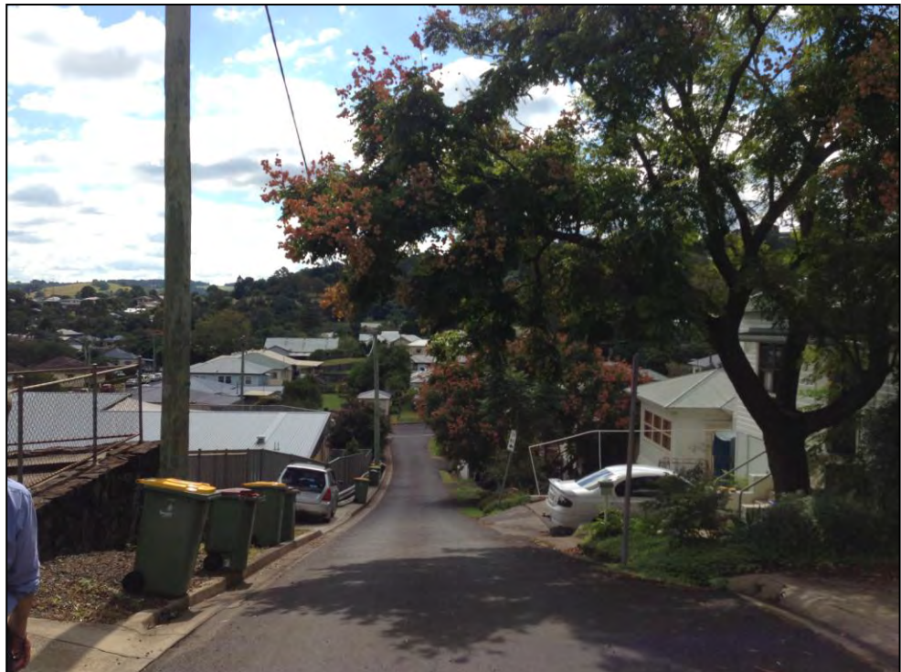
Photo 12 - View looking North along Little Uralba Street (standing further north than the previous photo).
