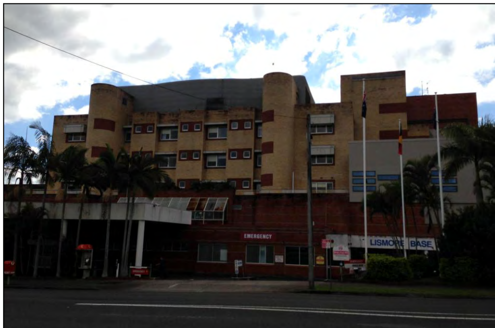
Photo 6 - Existing Main hospital entrance and emergency department (Block C) on Uralba Street.
