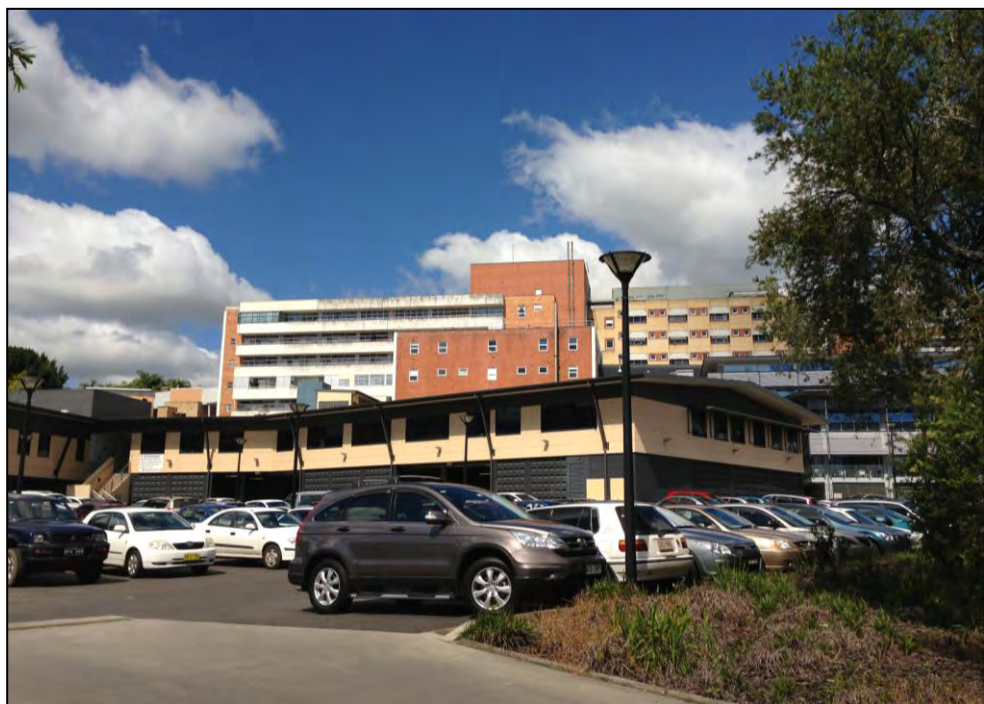
Photo 8 - View of LBH from the northern part of the site (Hunter Street) with the mental health unit in the foreground
