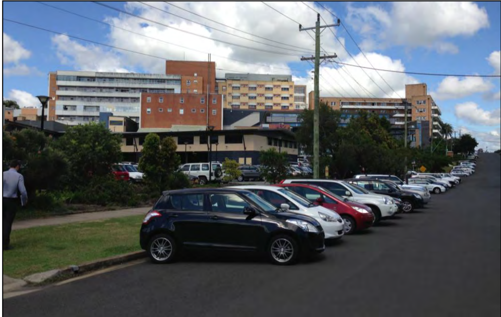
Photo 1 - View of the hospital from the northern part of Hunter Street, looking south/south-east Source: CPSD
