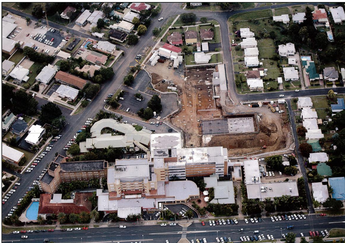
Figure 6.4: Excavation works as part of redevelopment planned in 1988. (Source: Courtesy of Owen Byrnes - Richmond Network Physical Resources Manager, NNSWLHD)
