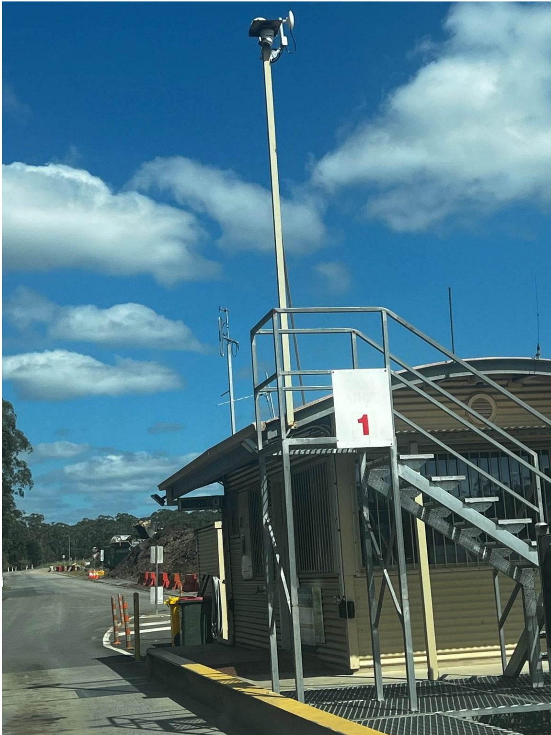
Weighbridge with inspection facilities.
