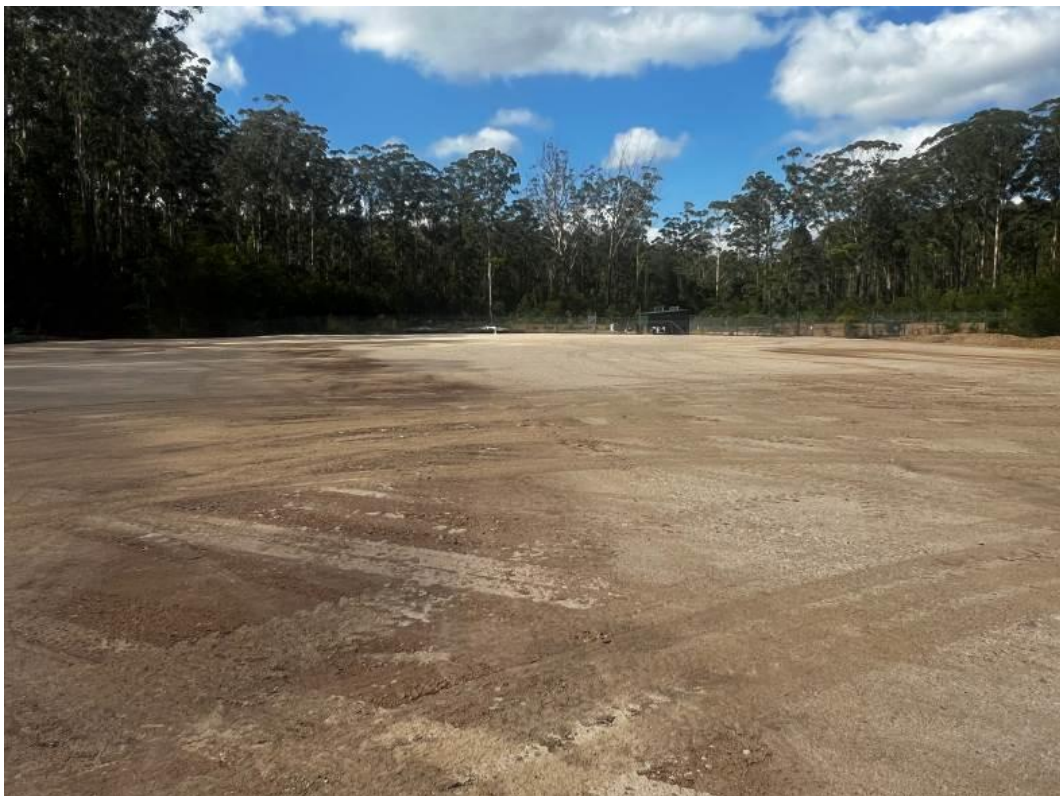
Construction for interim leachate collection tank pad as per Interim Leachate Management Plan.
