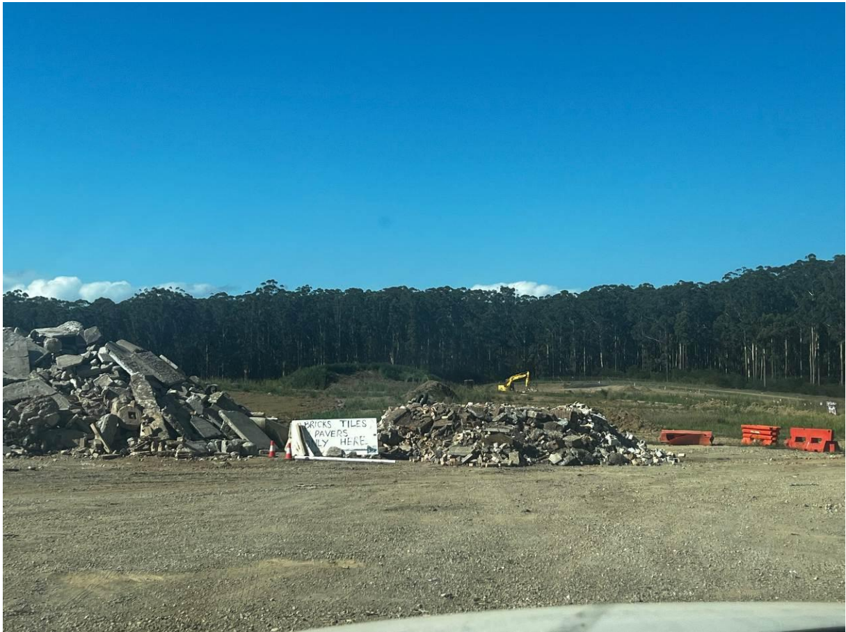
Waste separation – concrete, bricks, tiles & pavers.
