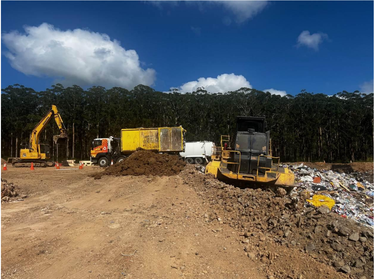
Tipping at active face.
