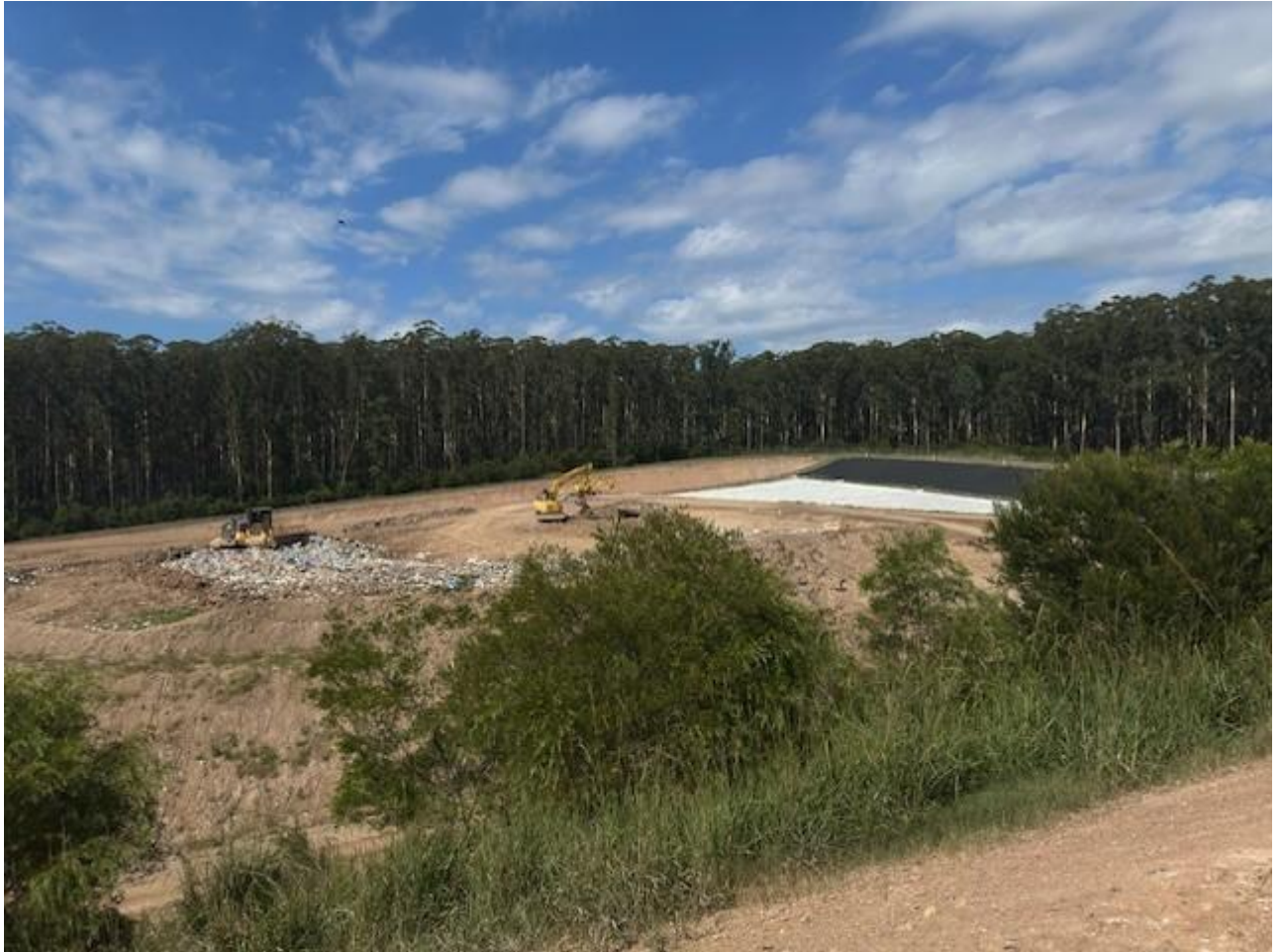
Stage 1 Landfilling Area.
