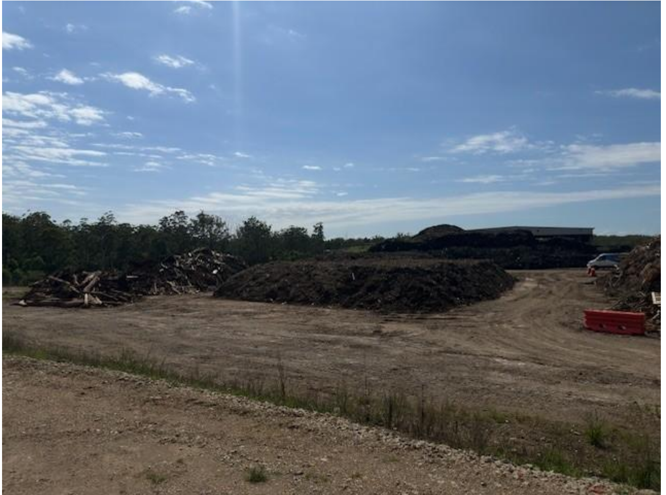
Organics Resource Recovery Facility.
