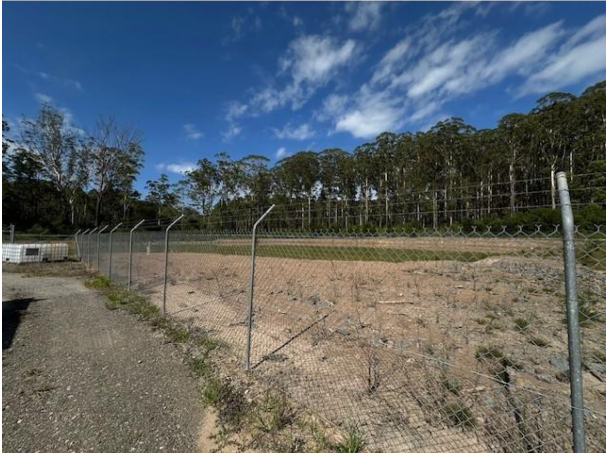
Fenced Sediment Pond.
