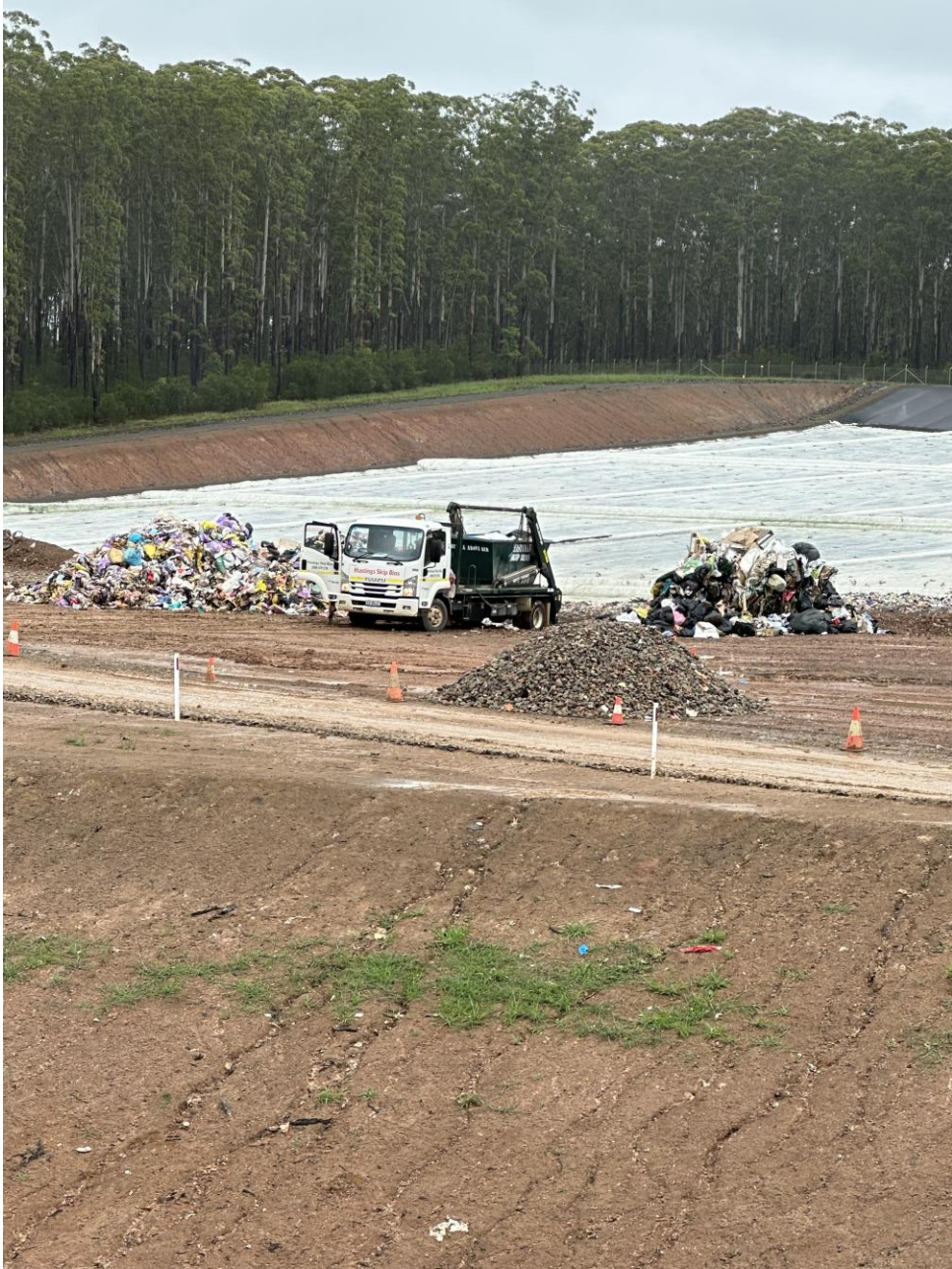
Landfilling in operation for fully lined Stage 1 cells
