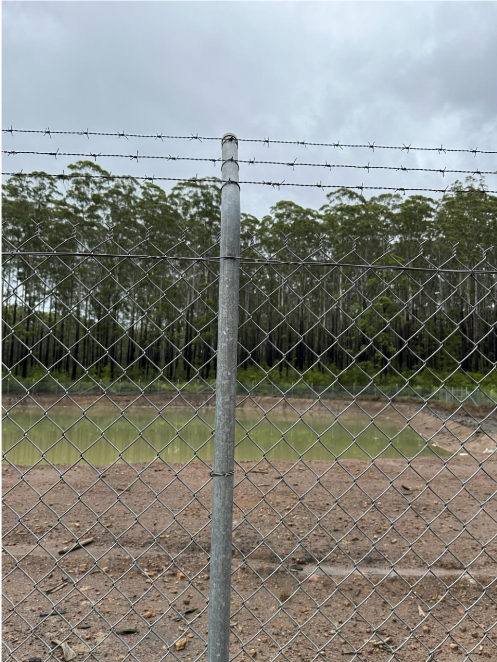
Fully fenced sediment pond
