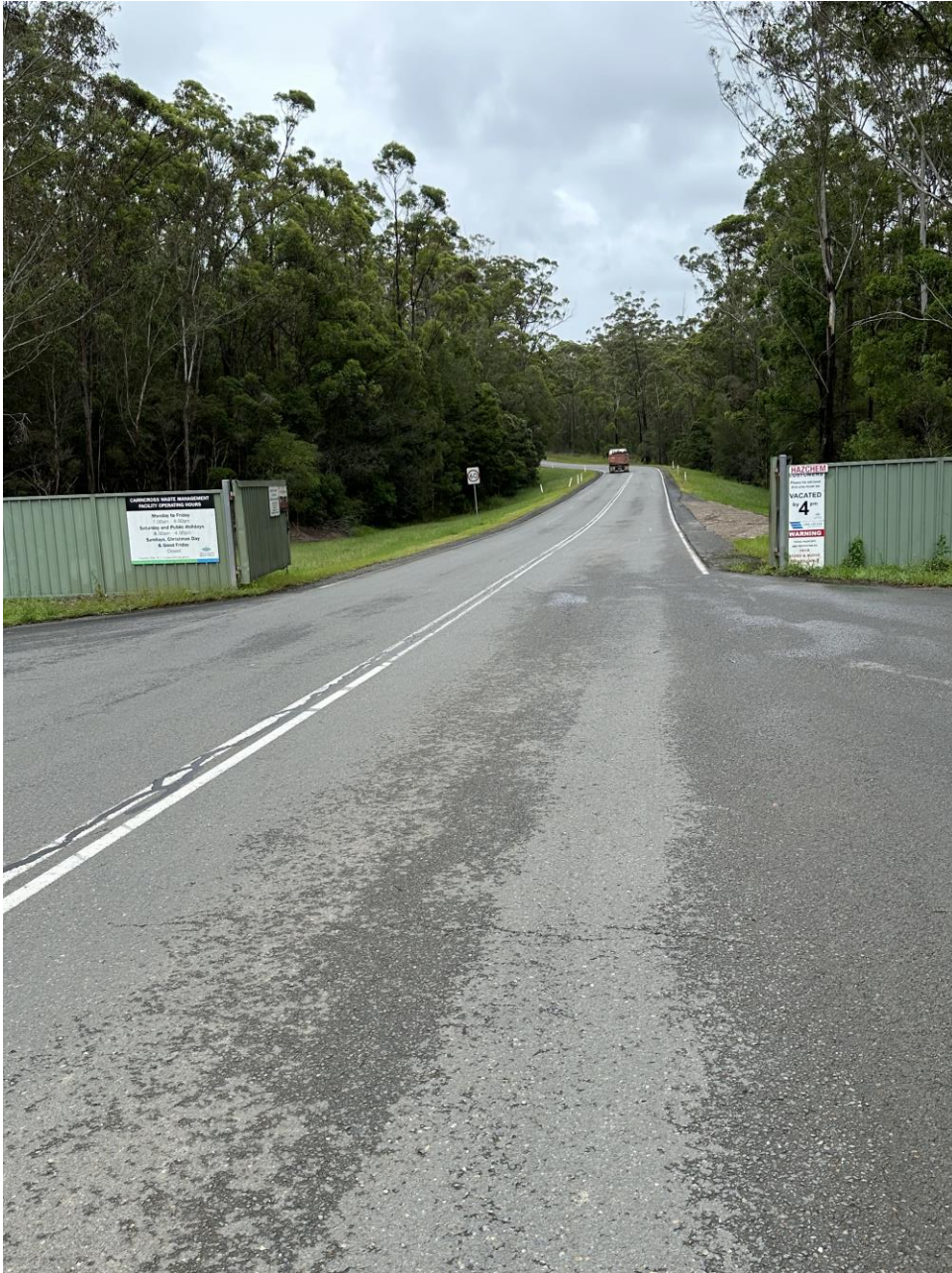
Approximately two kilometres site entrance with signages and contact details
