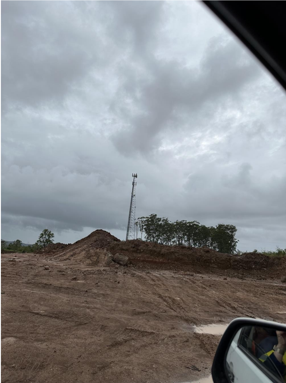
Excavated materials use for daily cover
