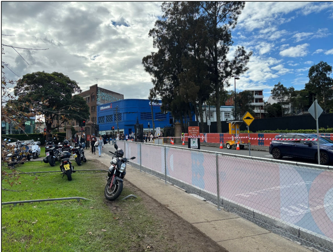
Figure 4 | Area on the western side of Western Avenue within the campus (Source: DPHI)
