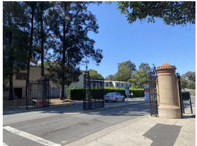
Figure 38 – Current demountable buildings, western façade and Ross Street gates, northern extent of subject site.
