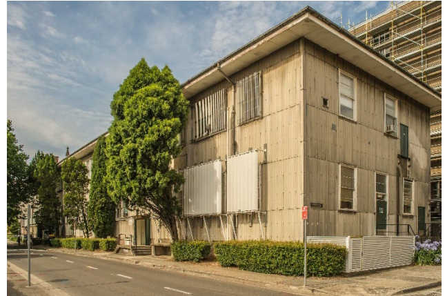
Figure 22 – The Transient Building, photographed in 2015 from Science Road.
