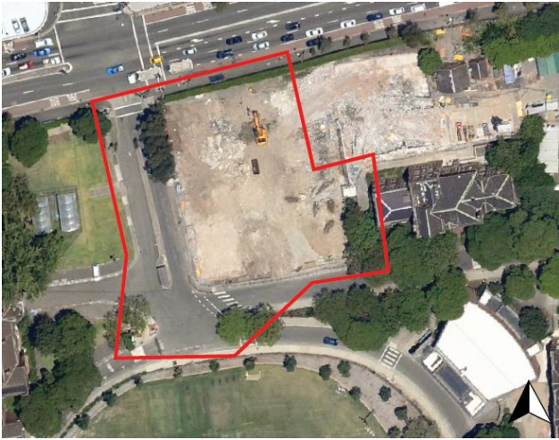
Figure 25 – The subject site in 2010, showing the demolition of the Transient Building.
