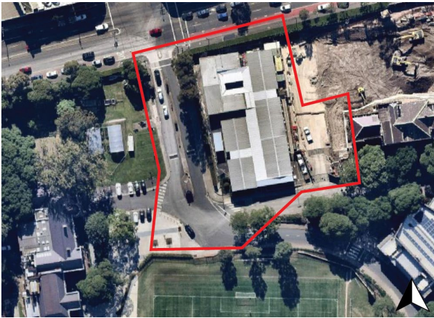
Figure 27 – The subject site in 2017, showing the current demountable building and demolition activity to the western extent.
