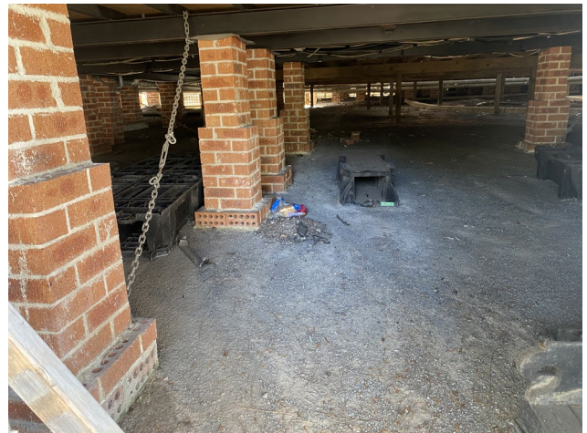
Figure 32 – View beneath current demountable buildings.
