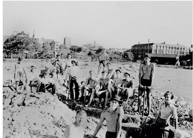
Figure 18 – University students photographed in the early 1940s engaged in the digging of campus air raid trenches.
