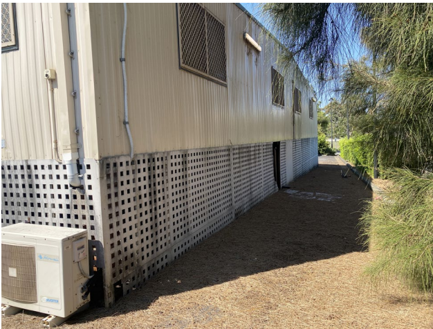
Figure 31 – Ground level of current demountable structures, north-western corner.
