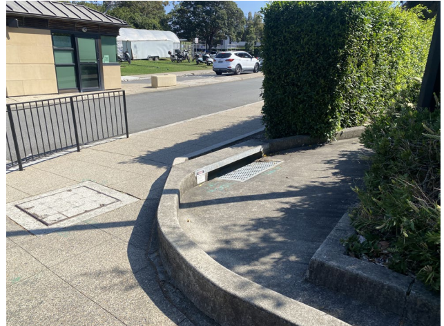
Figure 36 – Drainage infrastructure to pathing within the subject site, corner of Western Avenue and Science Road.
