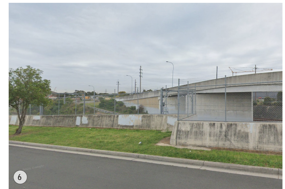
View of the proposed development from Wellington Road.
